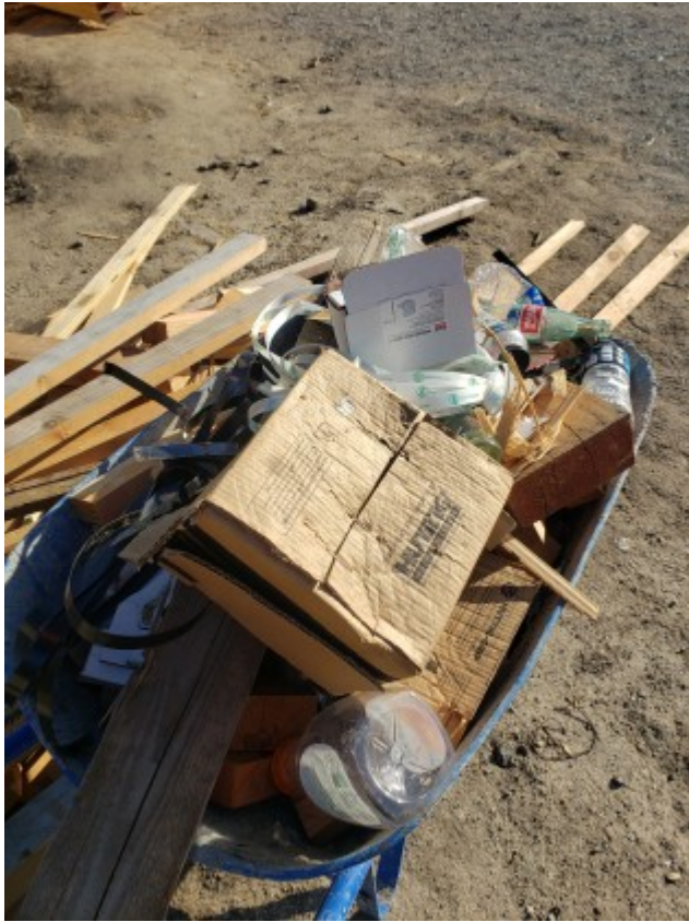
04/01/2021 - Food waste not placed in proper receptacle.
