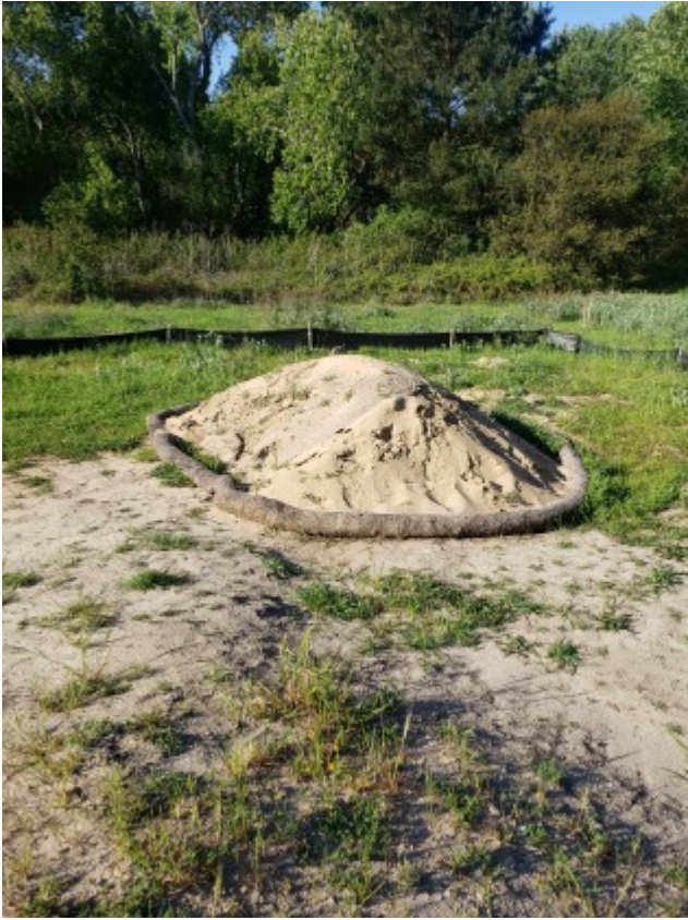
04/01/2021 - BMP insalled on soil stockpile.
