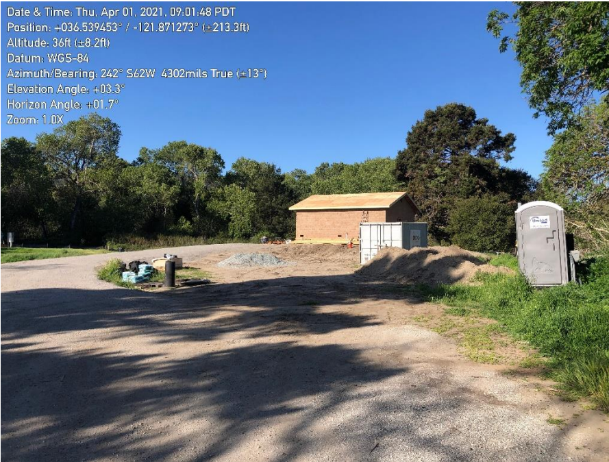
Photo 1. Pump station and overall site conditions.
