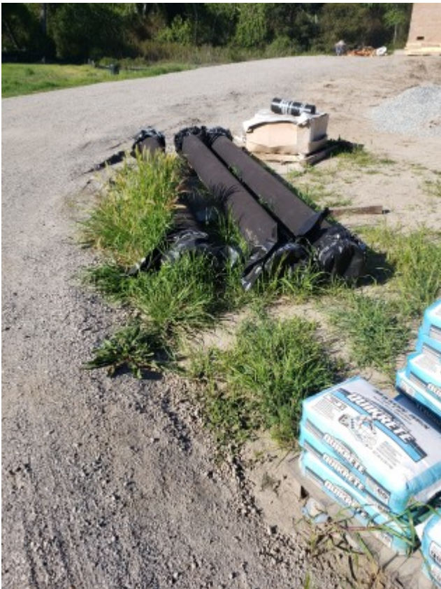
04/01/2021 - Piping on ground surface with covered ends to prevent wildlife entrapment.
