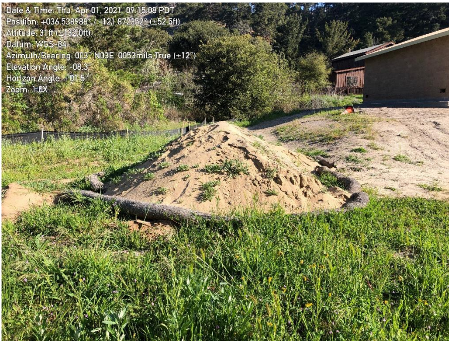
Photo 3. BMPs in place.
