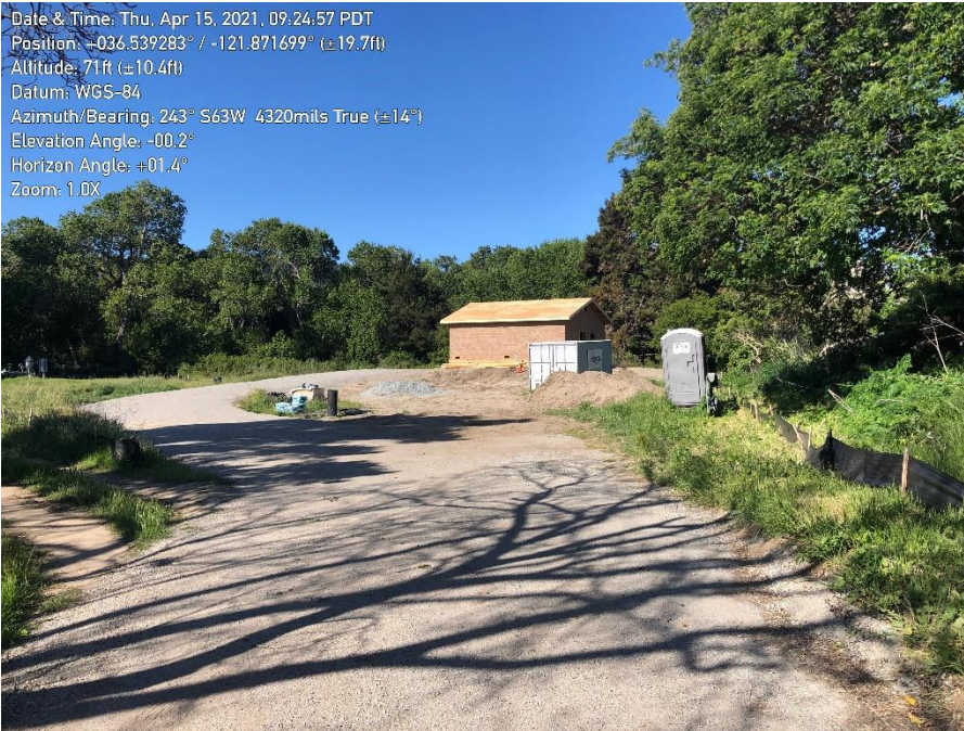
Photo 1. Pump station and overall site conditions.
