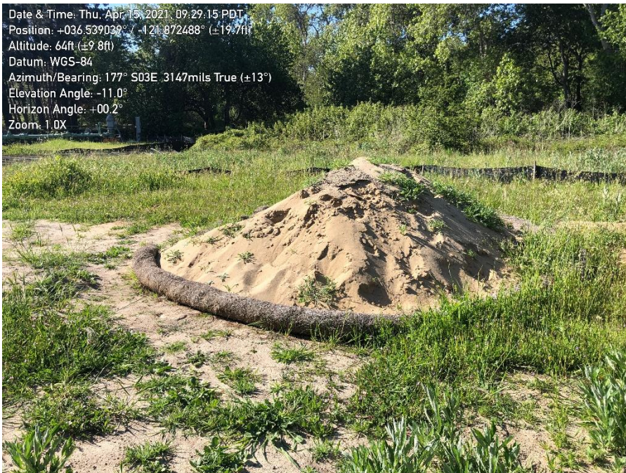
Photo 6. BMPs around stock pile.
