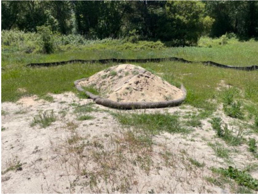
04/16/2021 - Existing straw wattle.
