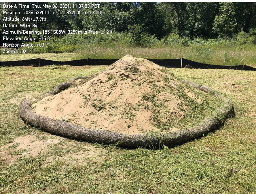
Photo 2. Spoils pile uncovered during weed removal activities. Monofilament straw wattle used.
