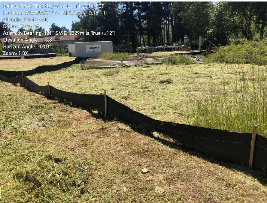
Photo 1. Mechanical weeding activities inside and outside of exclusion fence. Exclusion fence has been damaged by weed removal activities.
