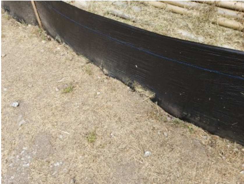
05/13/2021 - Exclusion fence to be repaired.
