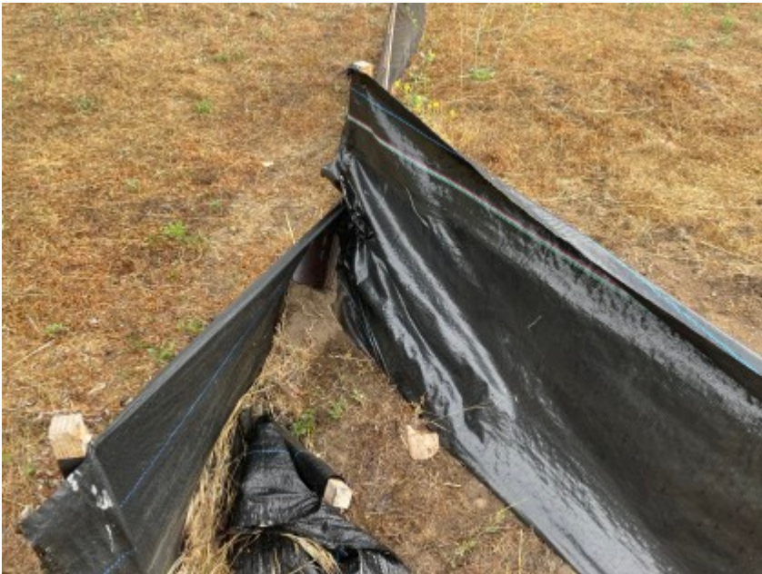
07/02/2021 - Open area in exclusion fencing needs to be filled.
