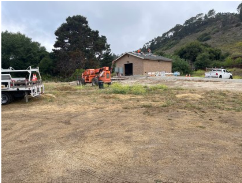
07/02/2021 - CVPS site conditions.
