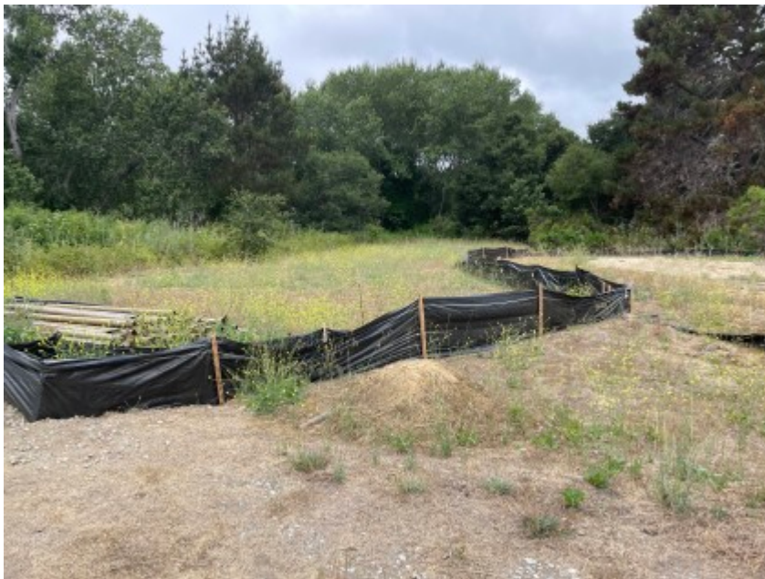
06/30/2021 - Intact exclusionary fencing on the southern border of CVPS.
