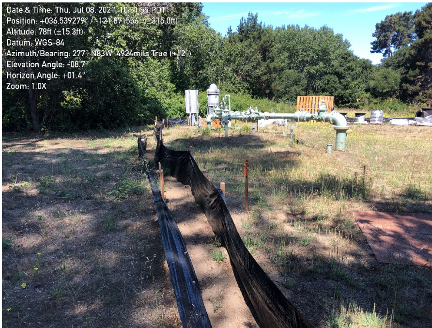
Photo 3. Silt fence in acceptable condition.
