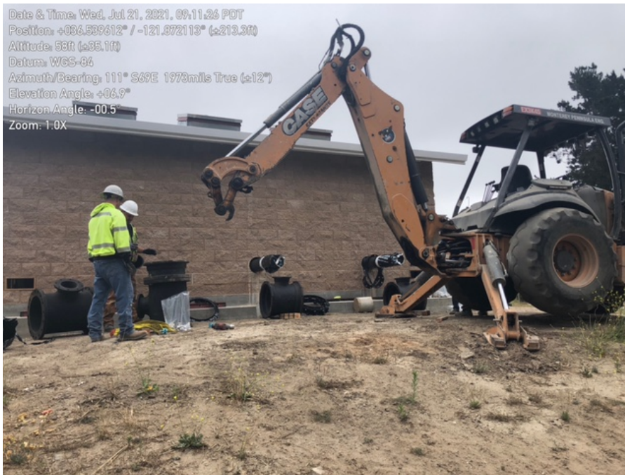
Photo 3. Preparing for pipeline installation on west side of pump station building.
