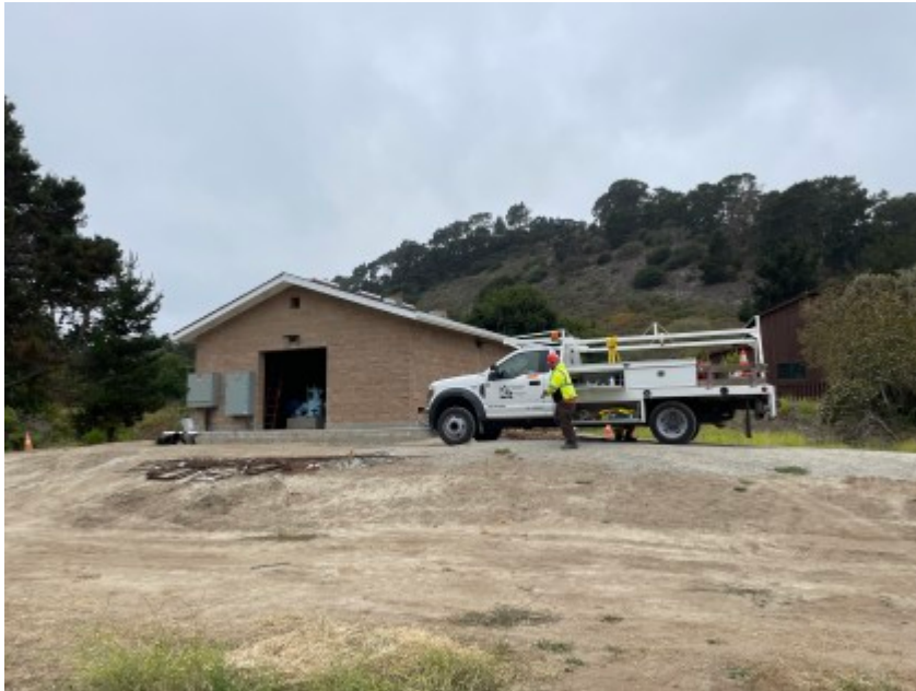
07/21/2021 - CVPS site conditions.
