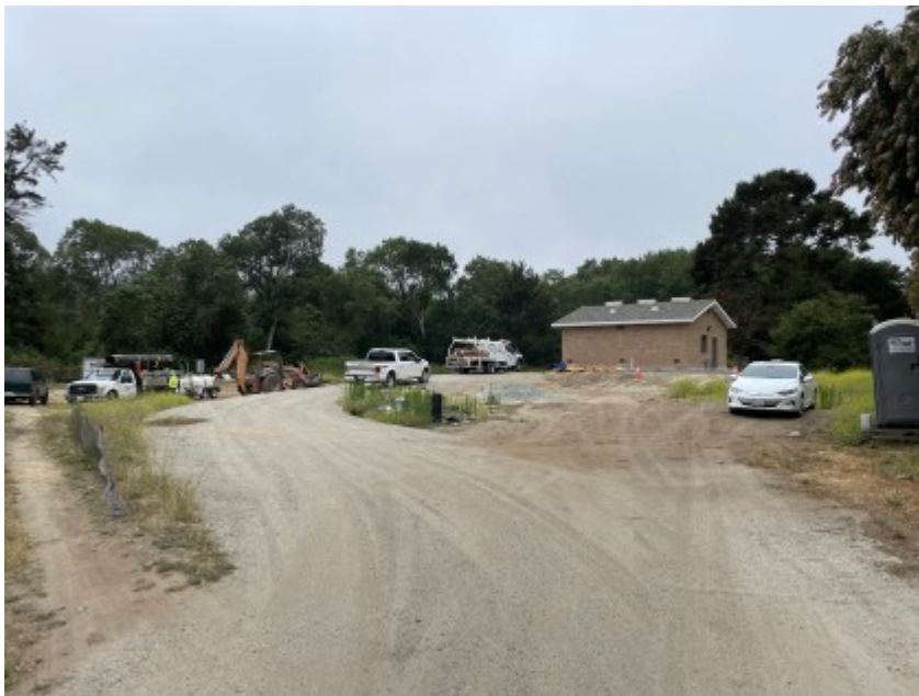
07/21/2021 - CVPS site conditions.
