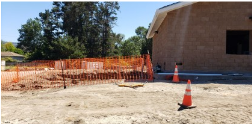
08/04/2021 - Fencing surrounding excavation.
