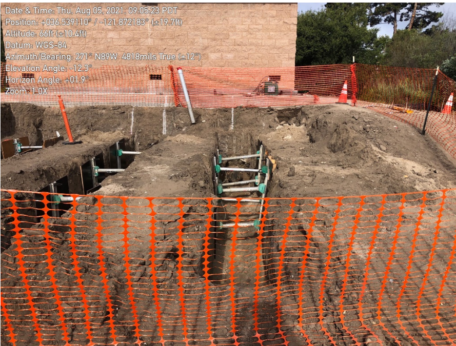
Photo 2. Trenches ramped to prevent wildlife entrapment.
