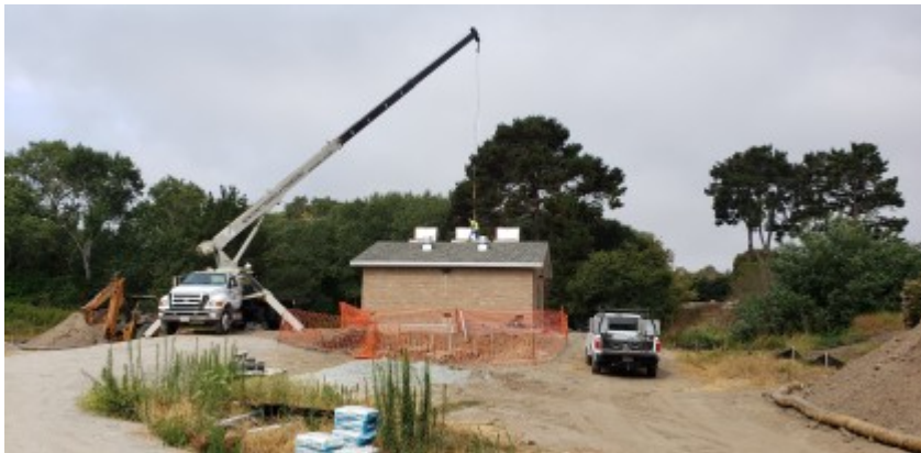
08/12/2021 - Installation of materials inside pump house.
