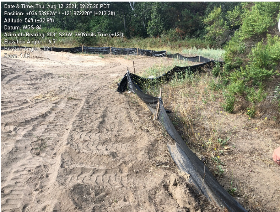
Photo 3. Silt fence in acceptable condition.
