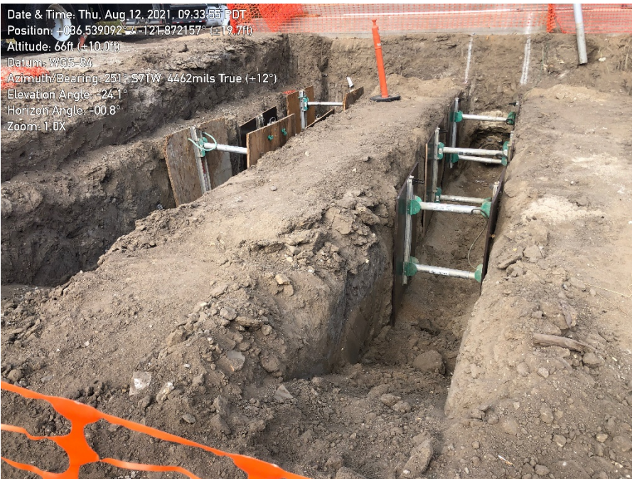
Photo 2. Trenches ramped to prevent wildlife entrapment.
