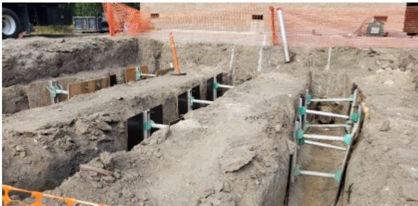
08/12/2021 - Trenches with wildlife escape ramps.
