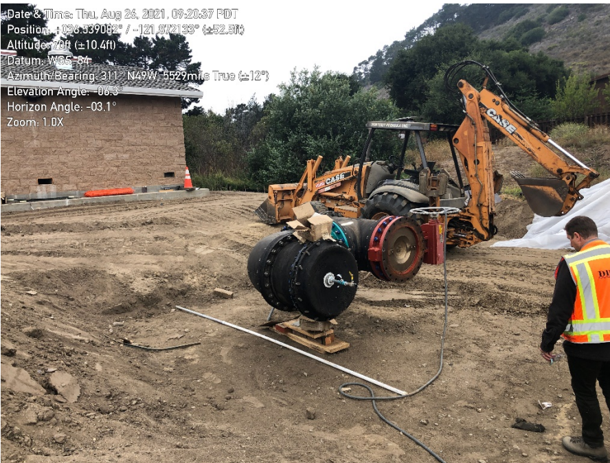
Photo 2. Trenches adjacent to pump station have been backfilled.
