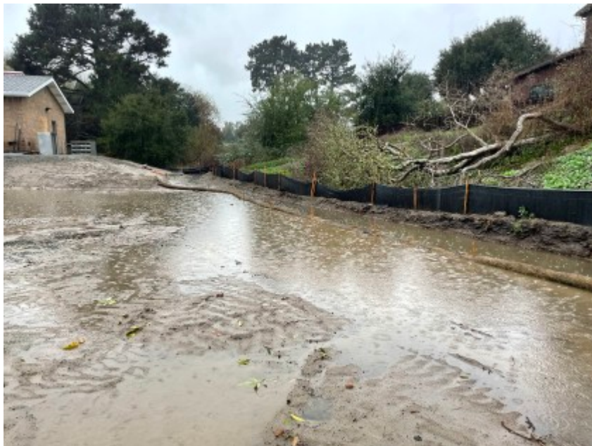
12/14/2021 - CVPS site conditions.
