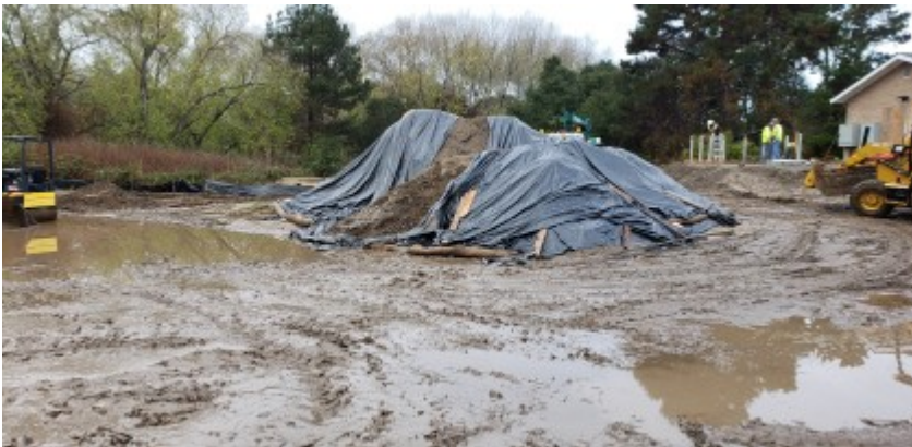
12/16/2021 - DD&amp;A recommended contractor repair spoils pile erosion control materials.
