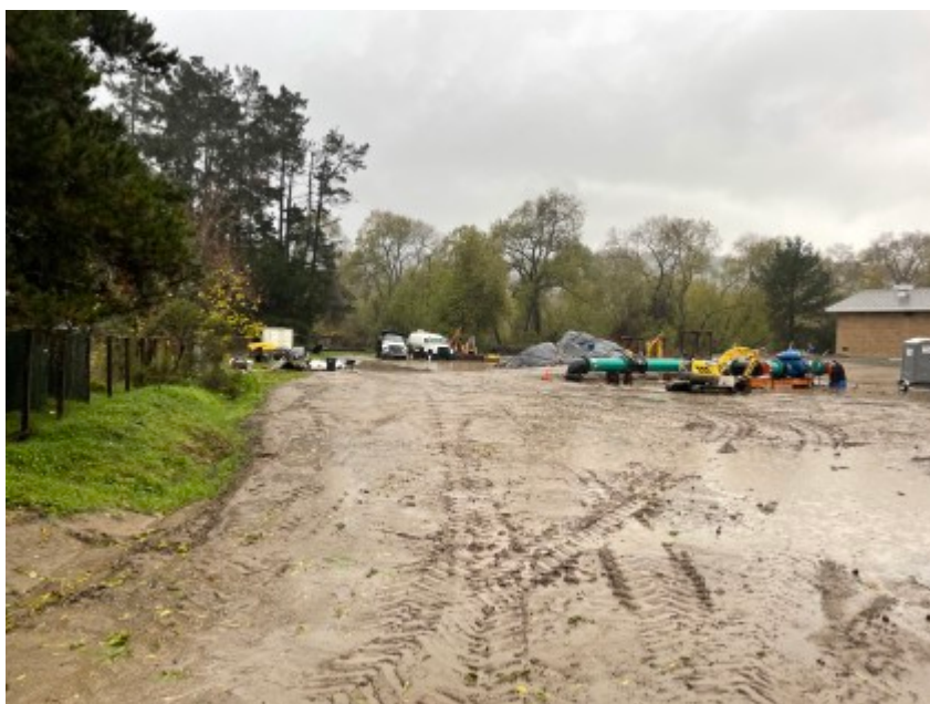
12/14/2021 - CVPS site conditions.
