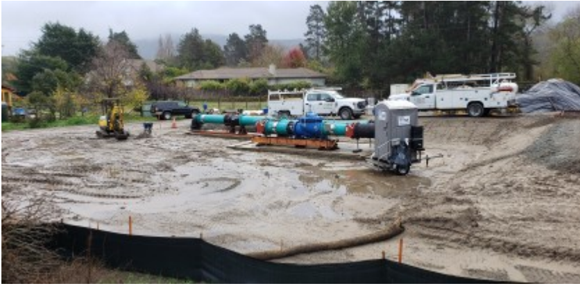
12/16/2021 - CVPS site conditions.
