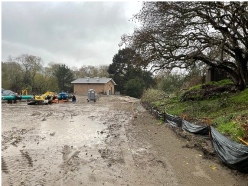
12/14/2021 - CVPS site conditions.
