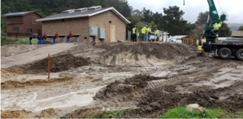
12/16/2021 - CVPS site conditions.
