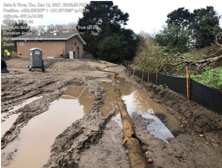
Photo 1. Monofilament straw wattle installed on site.
