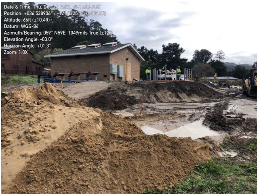
Photo 2. General site conditions.
