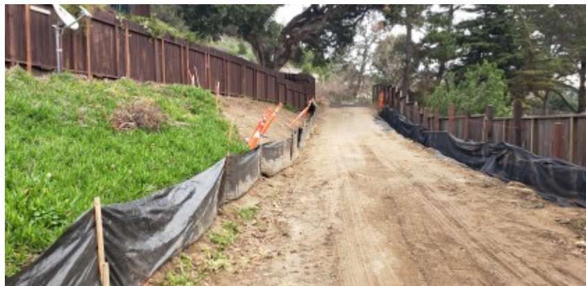
01/13/2022 - Exclusion fence reinstalled at site entrance.
