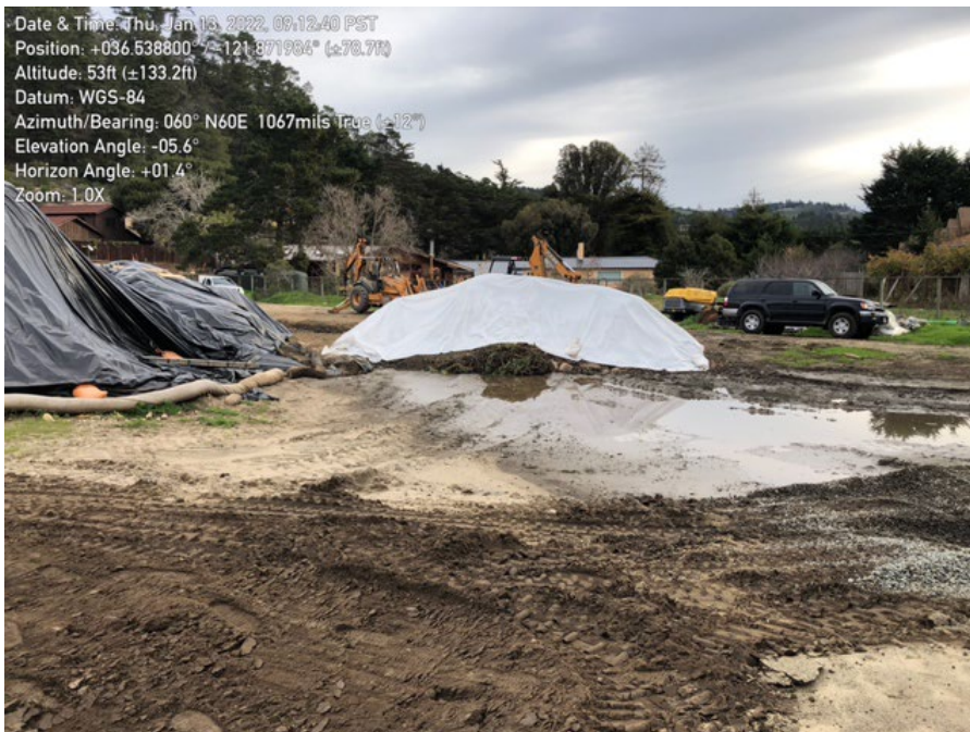
Photo 2. Spoils stock piles covered.
