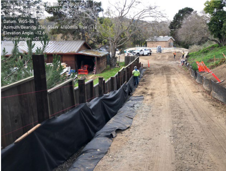
Photo 1. Retaining wall construction. Silt fence has been reinstalled along driveway.
