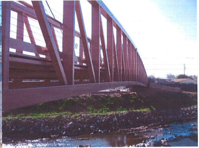
Lausett Ave Bridge - After!
