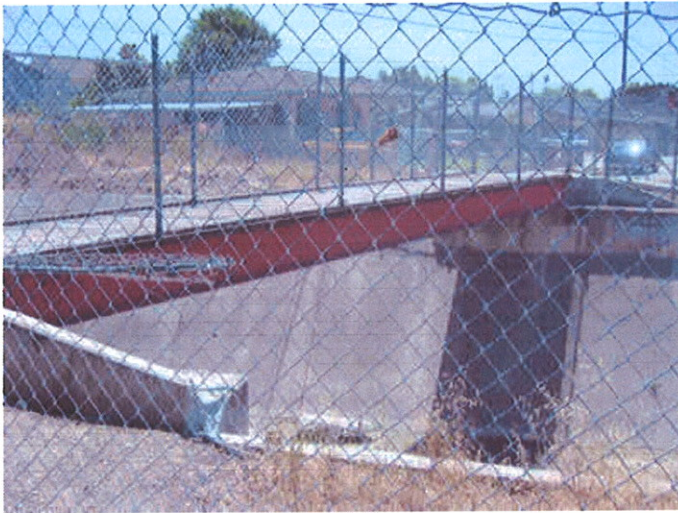
Lausett Ave Bridge - Before
