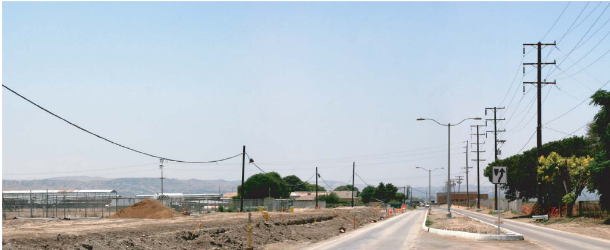
Existing Condition: Viewing west along Kimball Avenue
