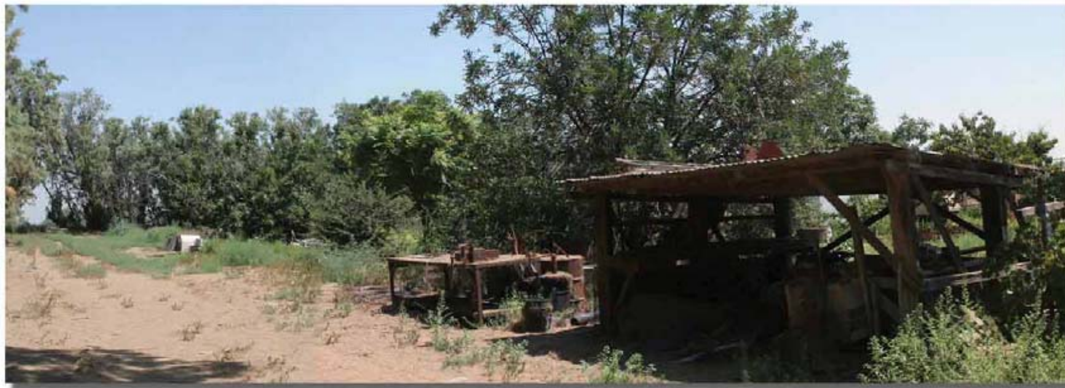
Existing Condition Photograph looking northeast
