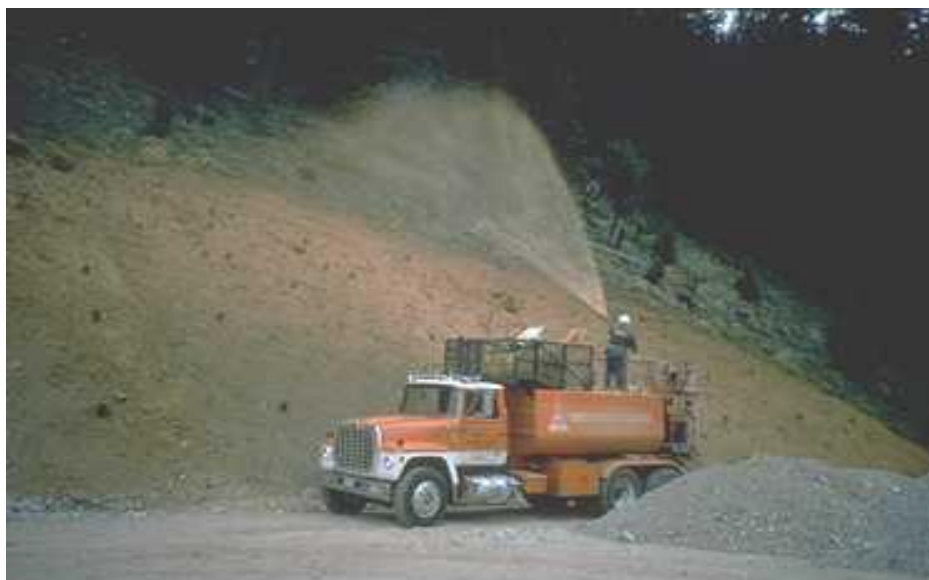
Applying hydraulic mulch.
