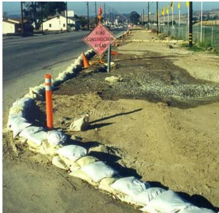
Sand bags used as perimeter control.
