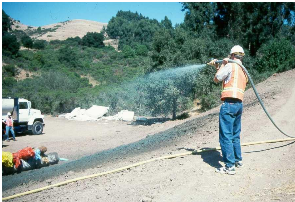
Applying hydroseed.
