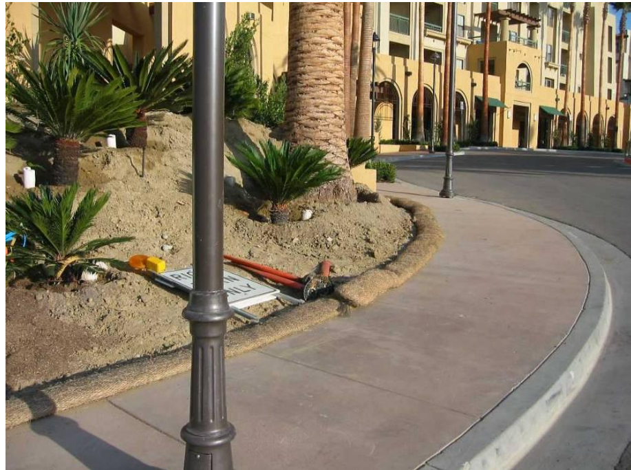
Fiber rolls as perimeter control.
