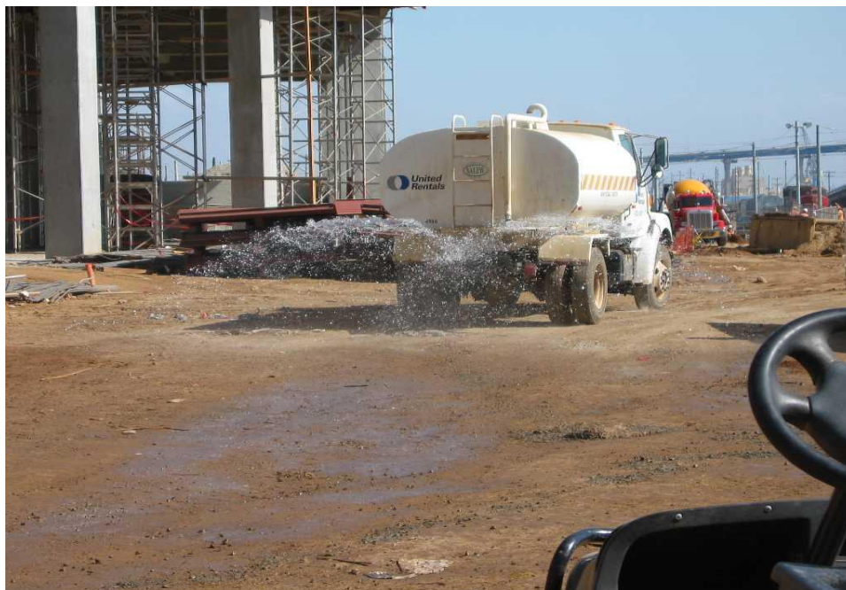
Water being applied for dust control.
