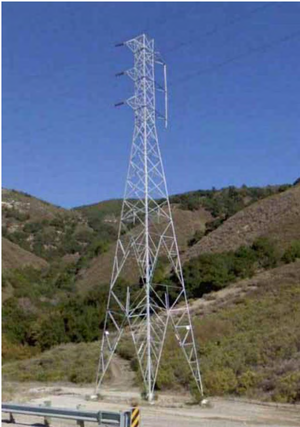
Figure 2.4-38: Typical Lattice Steel Tower
