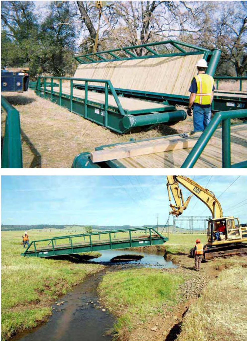
Figure 2.5-1: Typical Temporary Bridge
