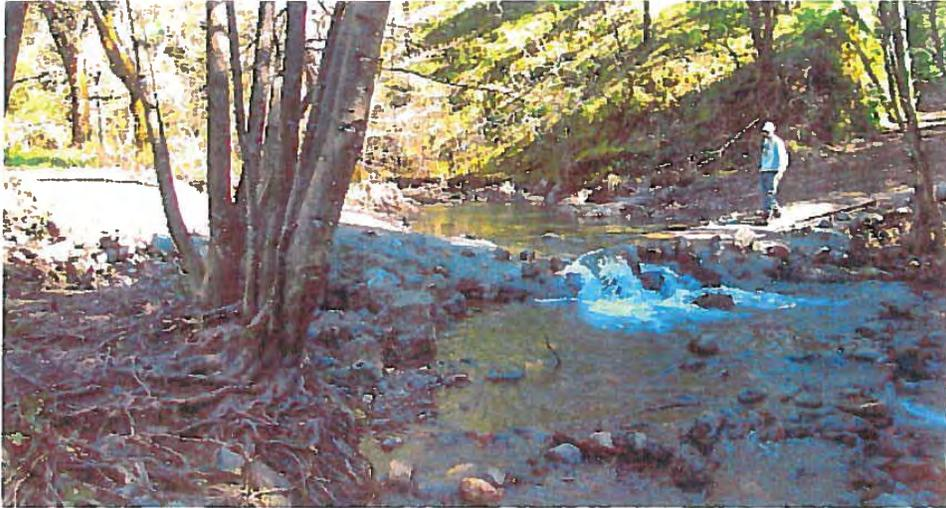
**FIGURE 122.** Wet ford on a Class II (non-fish) perennial stream.
