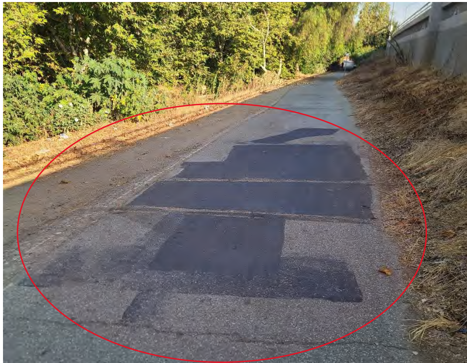
Figure 25. Various asphalt patching repairs, looking northwest
