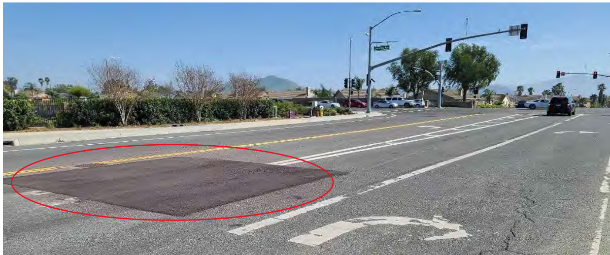
Figure 10 – Asphalt patch from previous utility work at the intersection of Pats Ranch Road and Limonite Avenue, looking southeast (March 2025)
