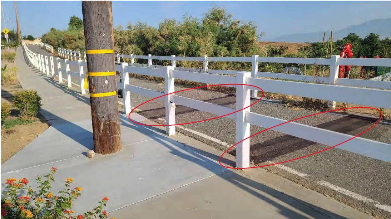
Figure 22. Trench repairs and missing wood fence on Santa Ana River Trail near the intersection of Jurupa Ave & Van Buren Blvd, looking northwest
