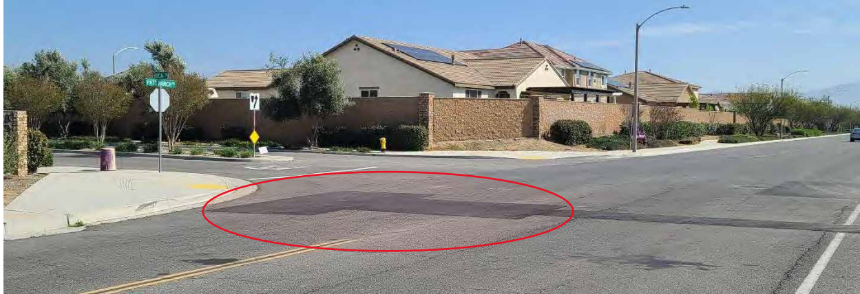
Figure 9 – Asphalt patch from previous utility work at the intersection of Pats Ranch Road and Boca Place, looking south (March 2025)
