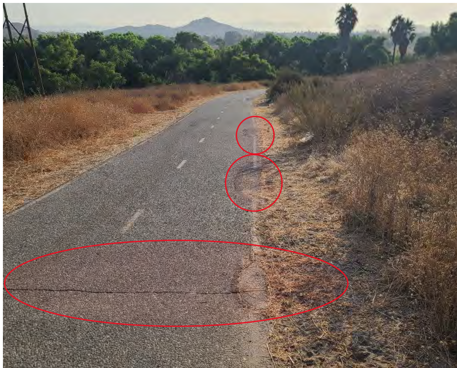
Figure 16. Santa Ana River Trail north of Jurupa Avenue with potholes and damage, looking northeast
