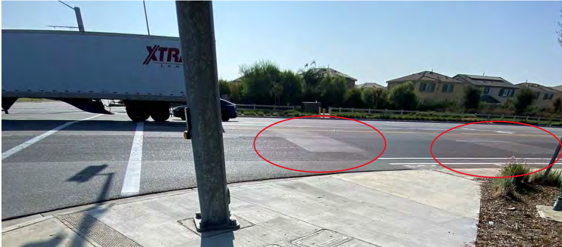
Figure 3 - Utility trench repairs observed at the intersection of Wineville Road and Cantu Galleano Ranch Road, looking southeast
