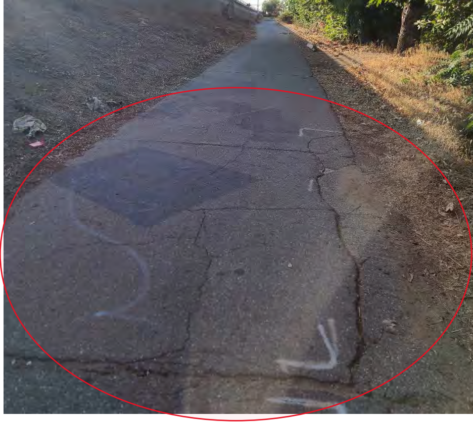
Figure 26. Asphalt cracking, patching repair and graffiti, looking southeast
