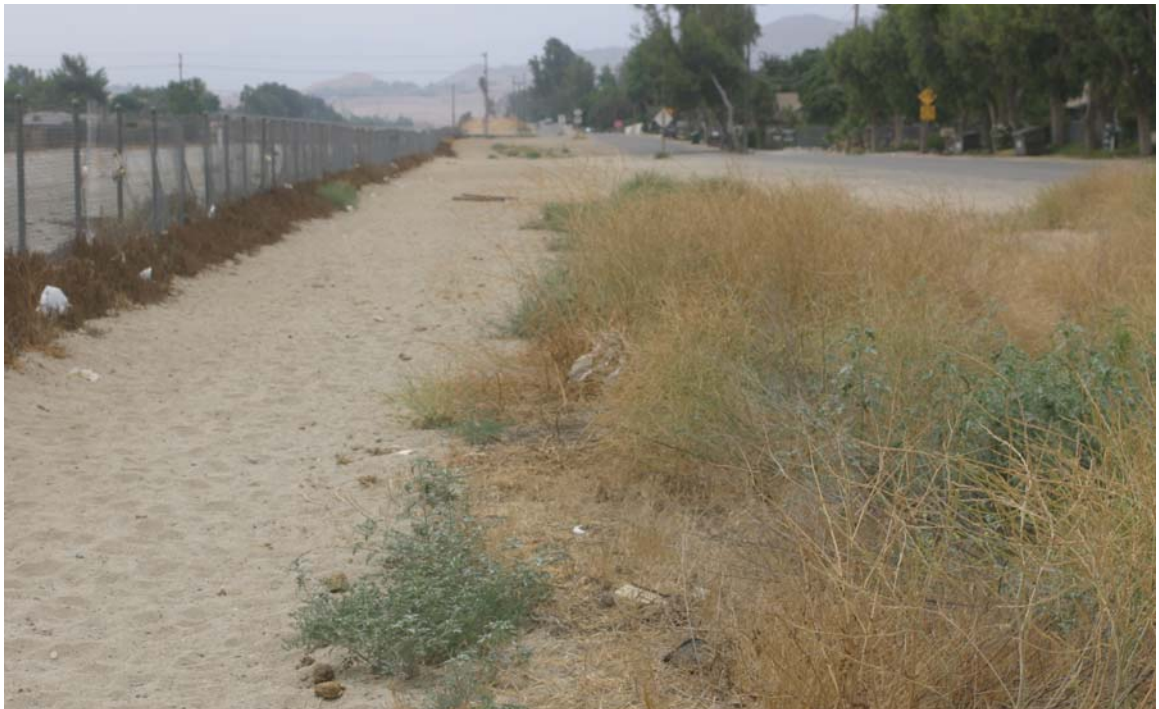
Figure 25. Photograph of the northern portion of survey Area 12, showing exposed sands along an equestrian trail. Conditions on this site range from low (disturbed sands at left for example) to moderate (such as vegetated areas as seen on the right).
