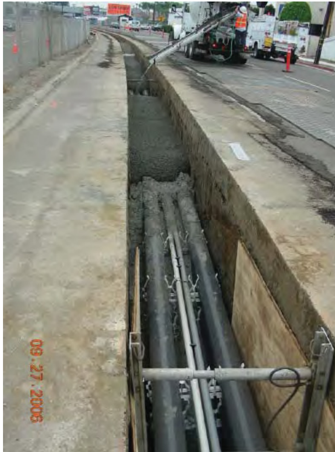
Figure 2: Example of Concrete Encased Duct bank
