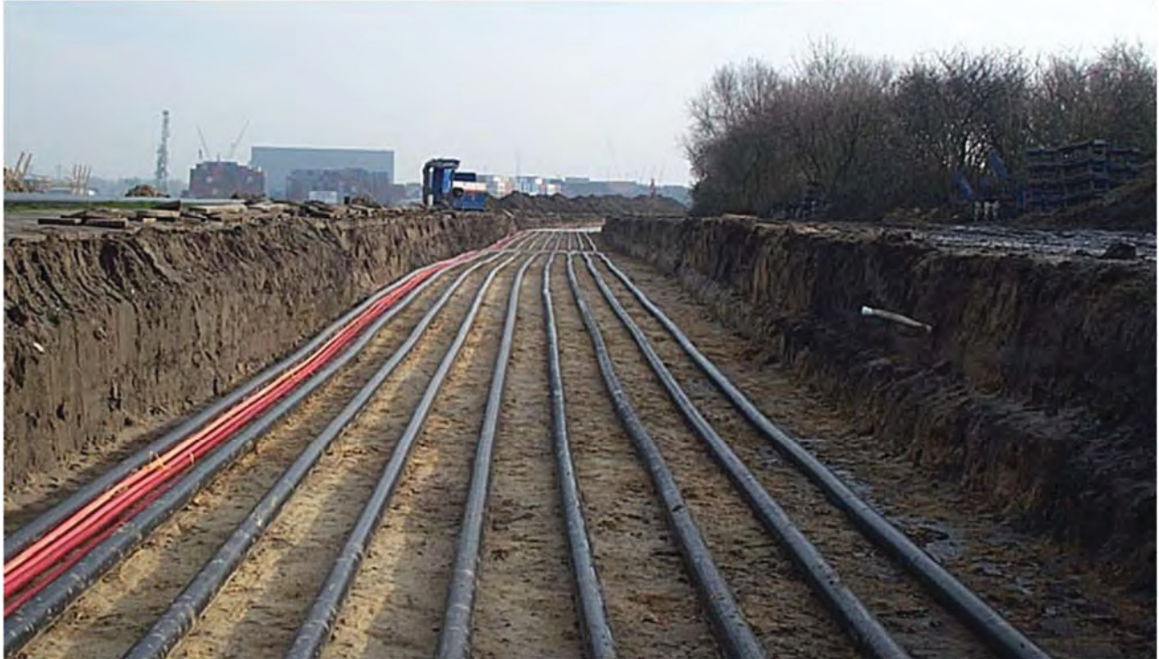
Figure 3: Example of Direct Buried Cable Installation
