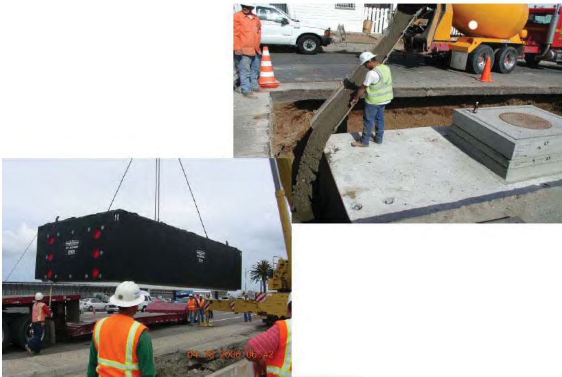
Figure 10: SDG&E 230 kV Vault Installation
