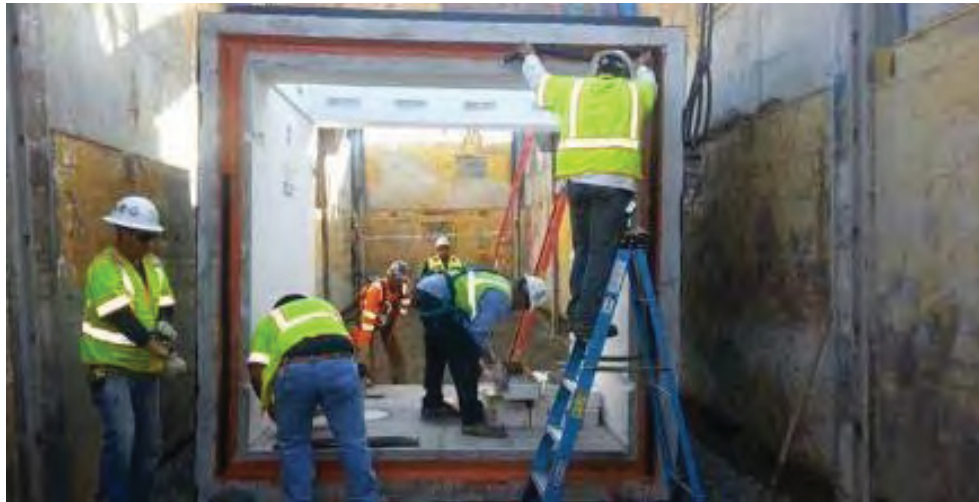
Figure 11: SCE 500 kV Vault Installation
