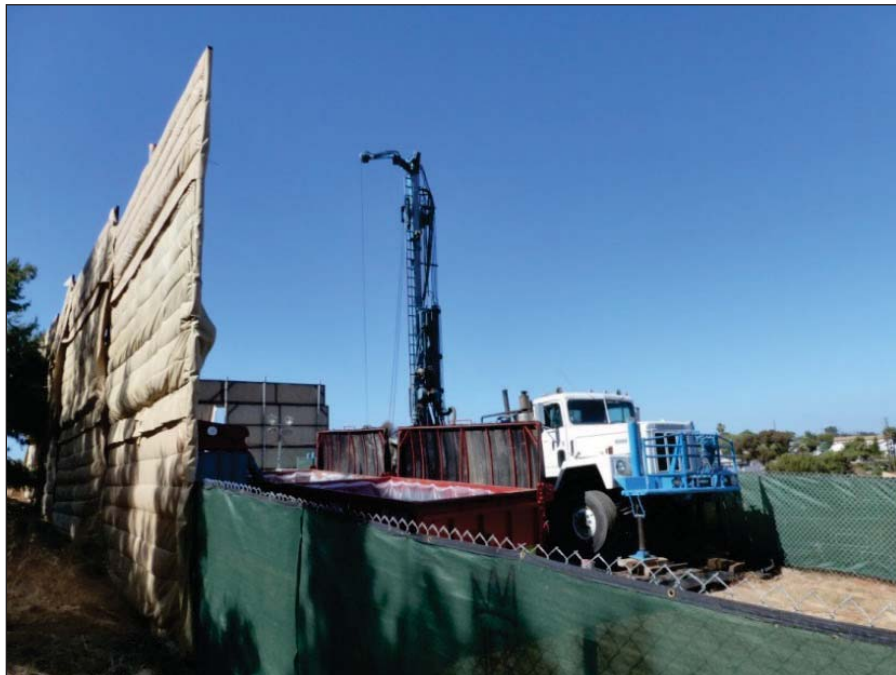
Figure 8 Sample Site-Erected Curtain-type Noise Barrier
