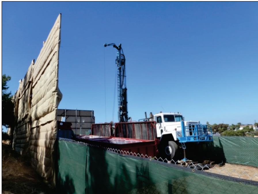
Figure 8 Sample Site-Erected Curtain-type Noise Barrier
