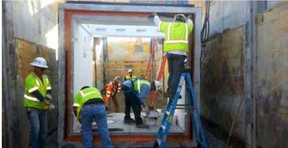
Figure 11: SCE 500 kV Vault Installation
