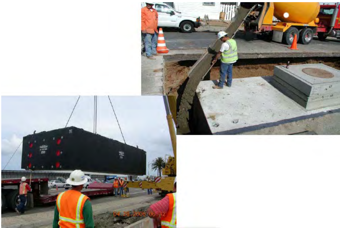
Figure 10: SDG&E 230 kV Vault Installation
