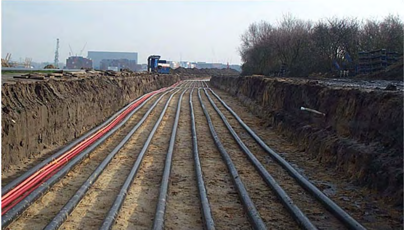
Figure 3: Example of Direct Buried Cable Installation
