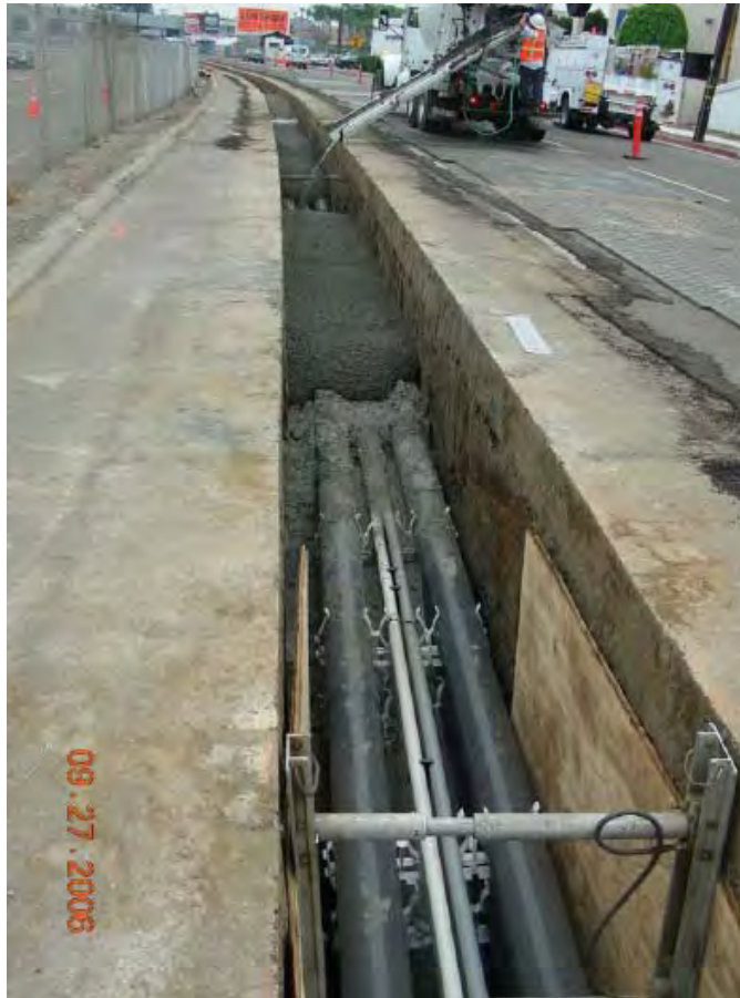
Figure 2: Example of Concrete Encased Duct bank
