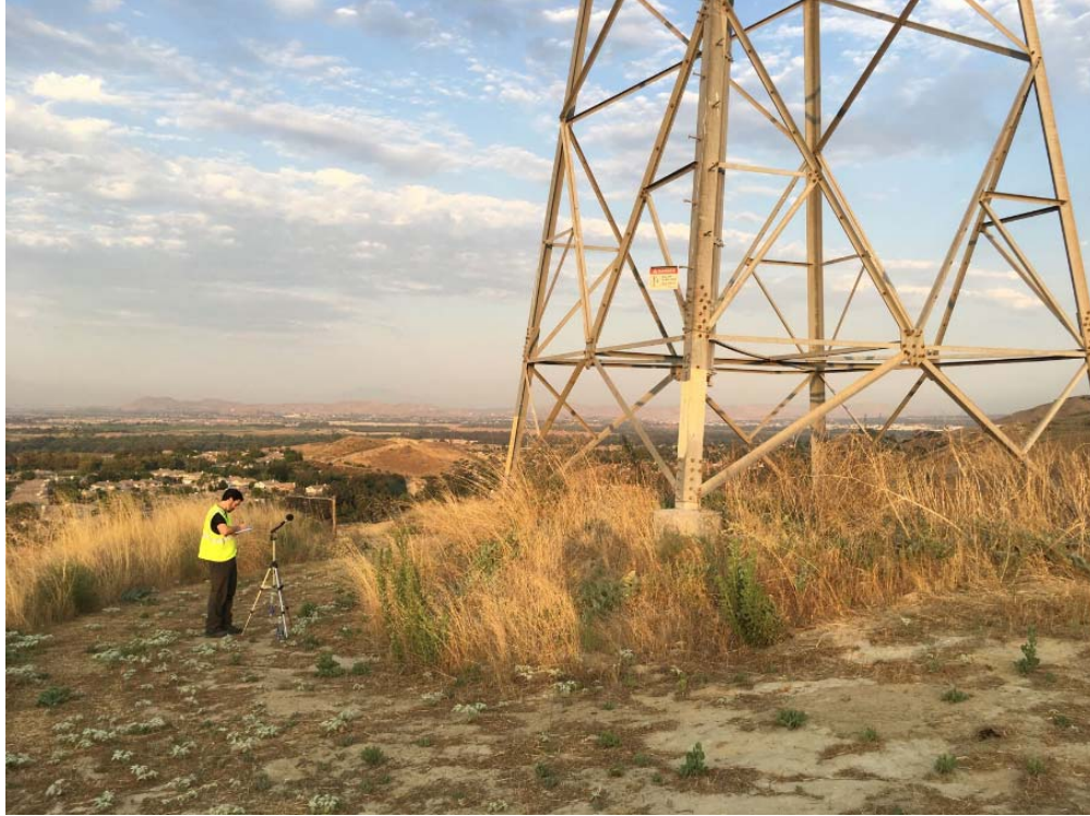
View from the west of the corona noise measurement location (facing east)
