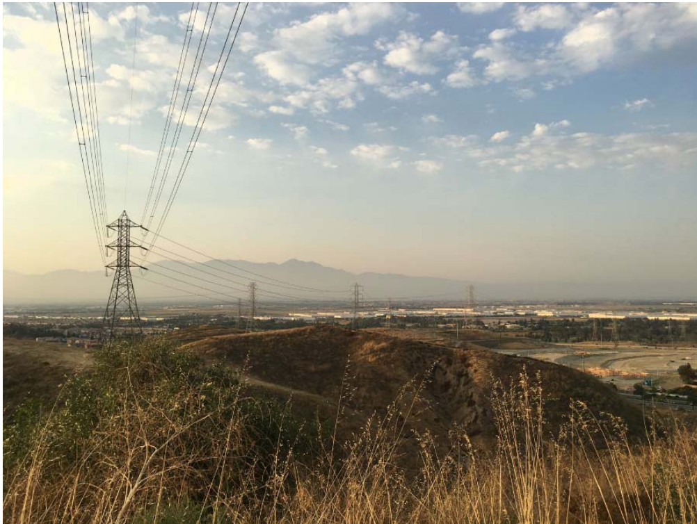
View from the south of the corona noise measurement location (facing north)
