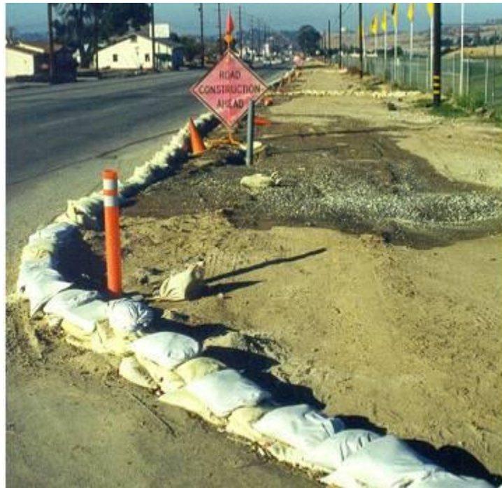
Sand bags used as perimeter control.
