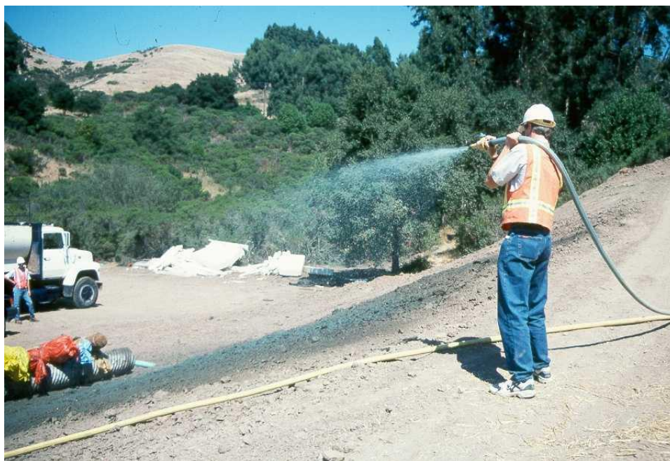
Applying hydroseed.
