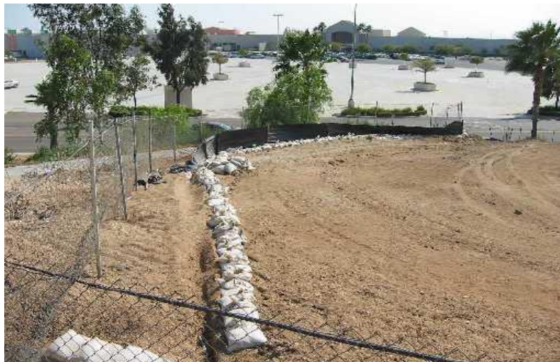
Gravel bags used as perimeter control.
