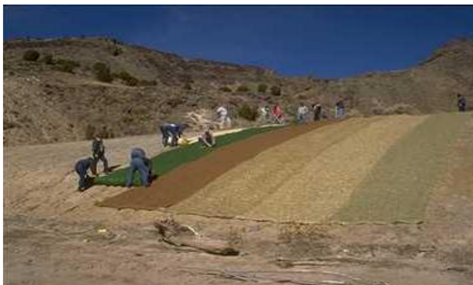
Several types of erosion control blankets.
