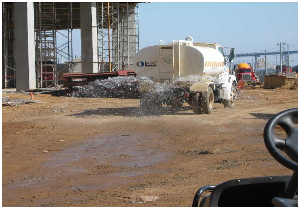
Water being applied for dust control.
