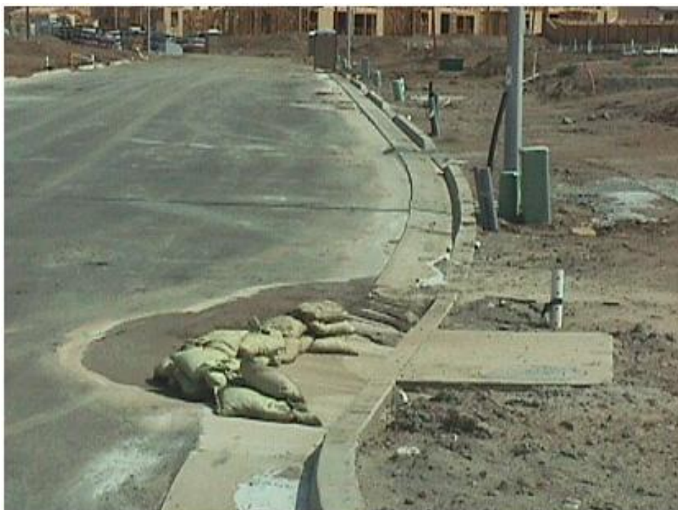
Gravel bag inlet protection.
