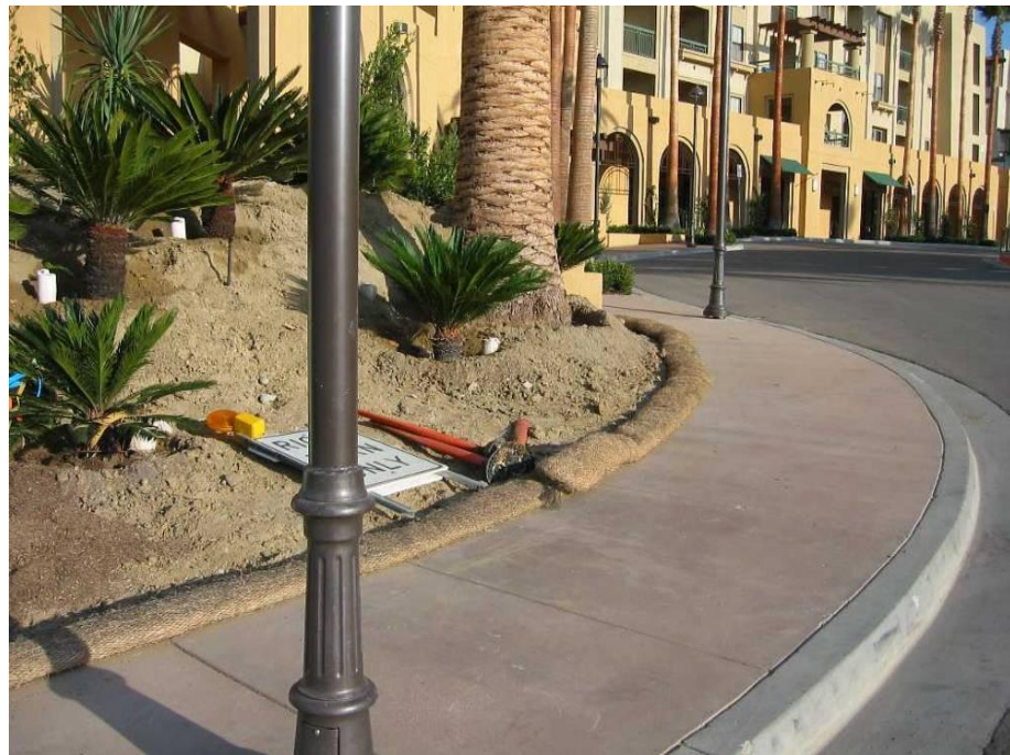
Fiber rolls as perimeter control.
