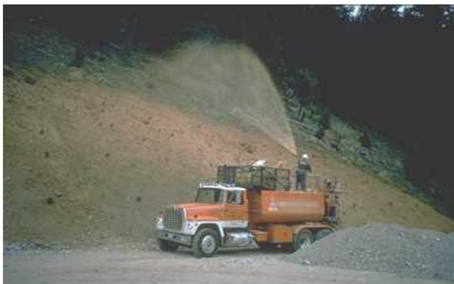
Applying hydraulic mulch.
