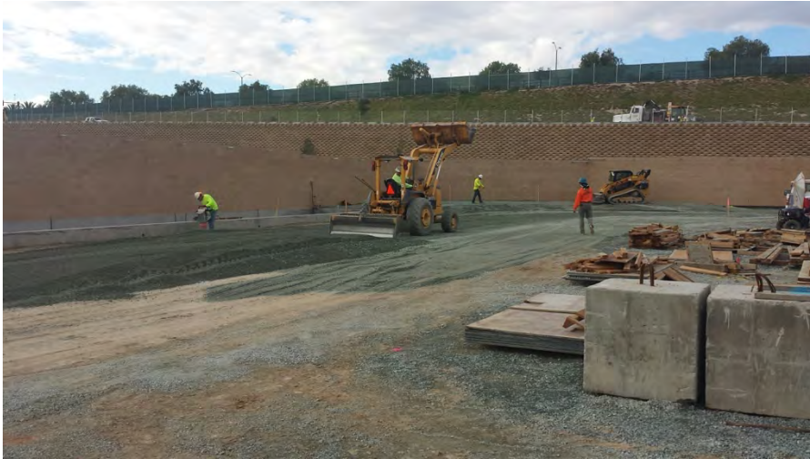
Photograph 1: Substation grading and base installation occurred during the week of December 19, 2016.
