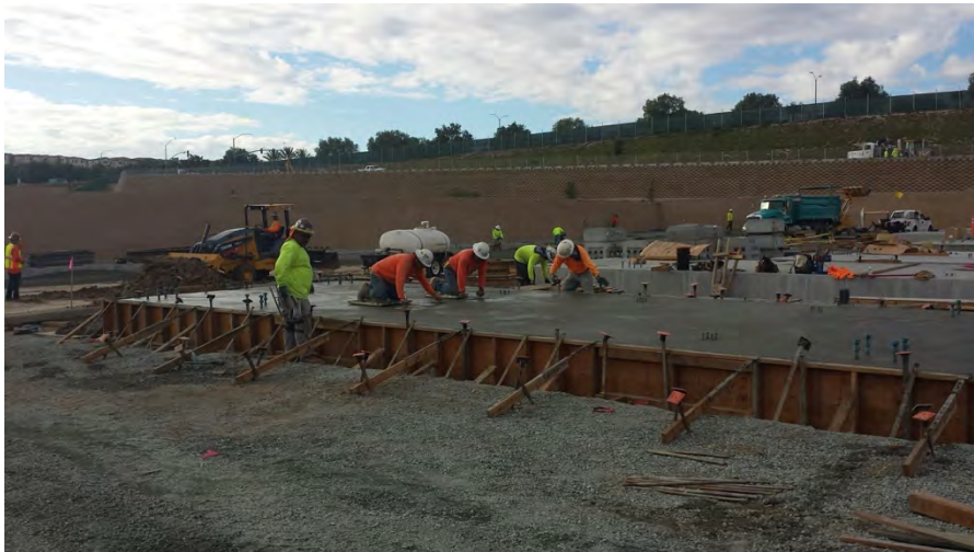
Photograph 2: Pouring and finishing concrete for substation equipment pads occurred during the week of December 19, 2016.
