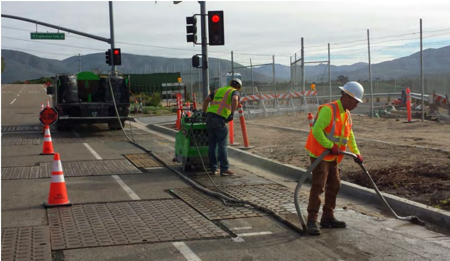
Photograph 1: Saw-cutting the pavement on Hunte Parkway for curb and gutter installation occurred the week of February 25, 2017.
