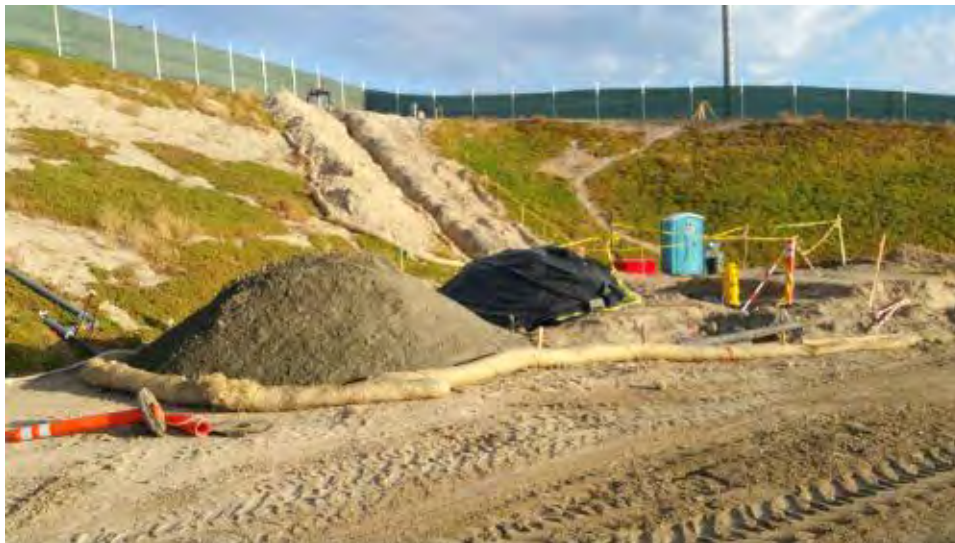
Caption Temporary BMPS below open trench for water line.
