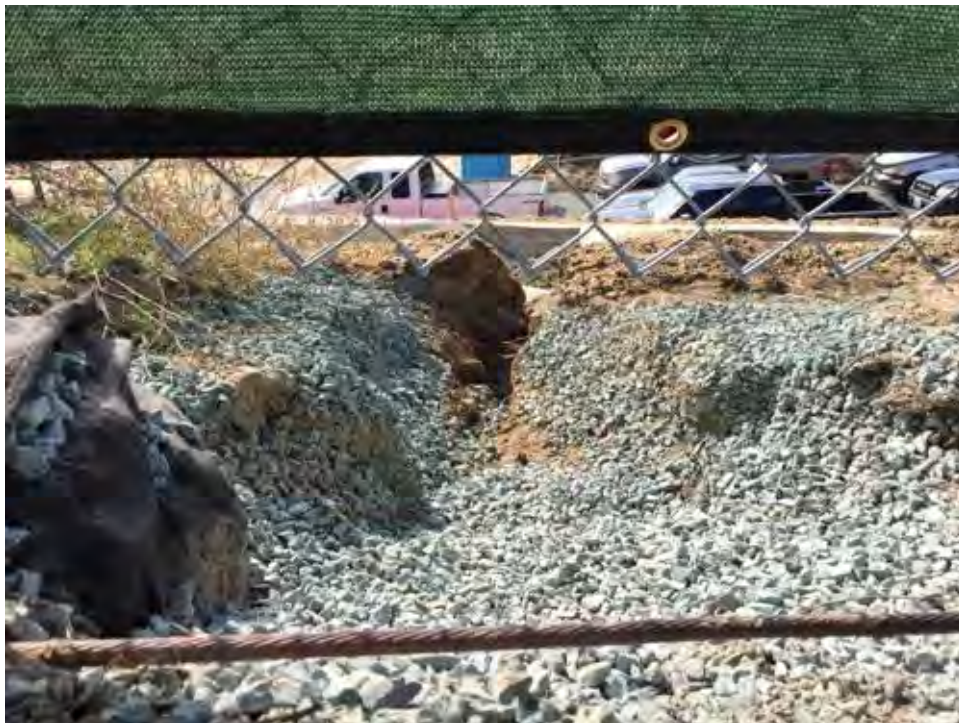
Caption Erosion above brow ditch from gully. Photo Attributes Capture Date/Time: Thu Dec 01 2016 11:42:37 GMT-0800 (PST)
