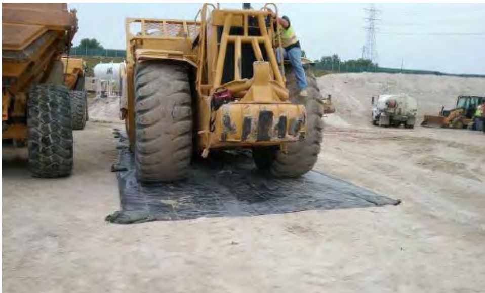
Caption Visqueen sheet beneath inactive equipment.
