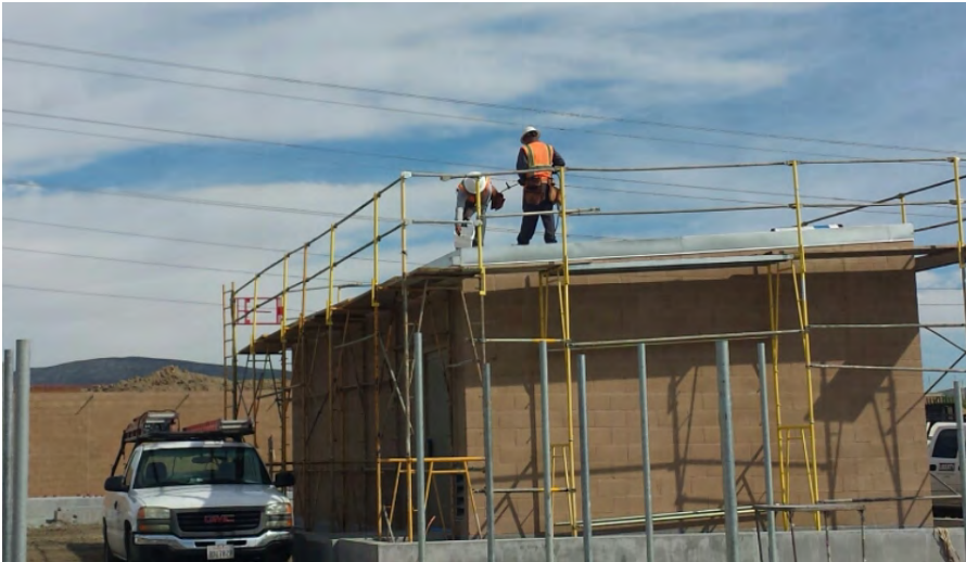
Photograph 2: Installation of the substation control-shelter roof occurred during the week of February 10, 2017.
