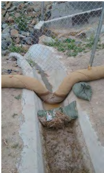
Caption Erosion control BMPs effectively capture runoff.
