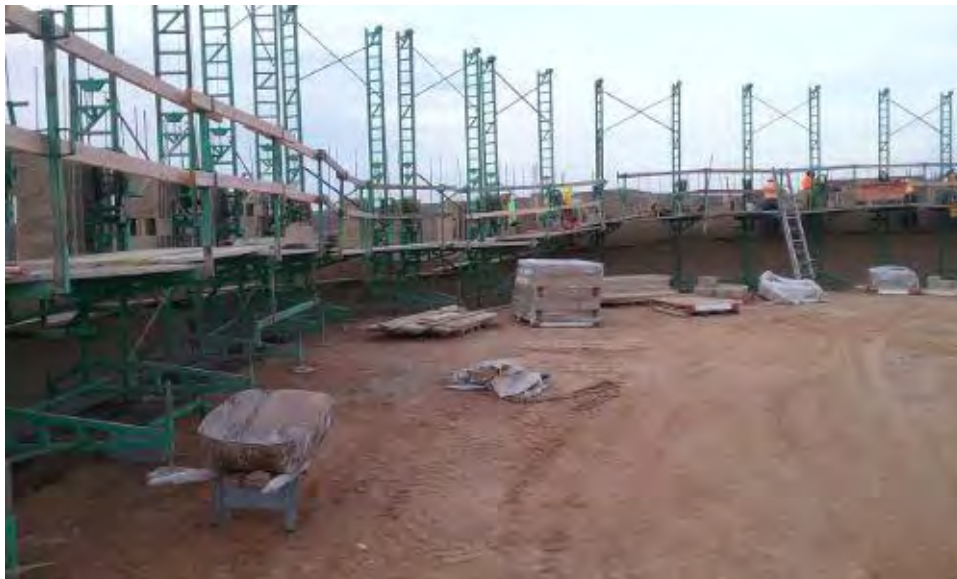
Caption Masonry screening wall construction.
