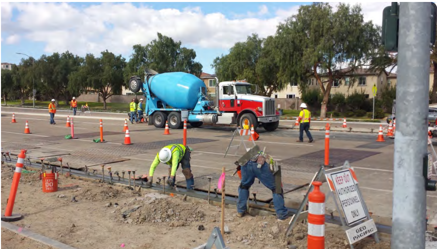
Photograph 2: Hunte Parkway curb and gutter concrete pouring occurred during the week of February 25, 2017.
