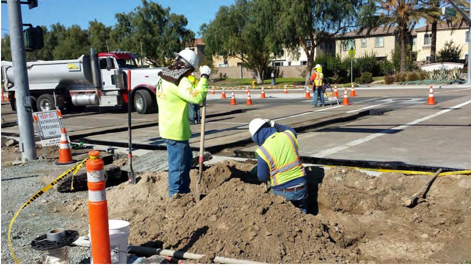
Photograph 3: Pot-holing to locate irrigation lines in Exploration Falls driveway occurred the week of March 04, 2017.
