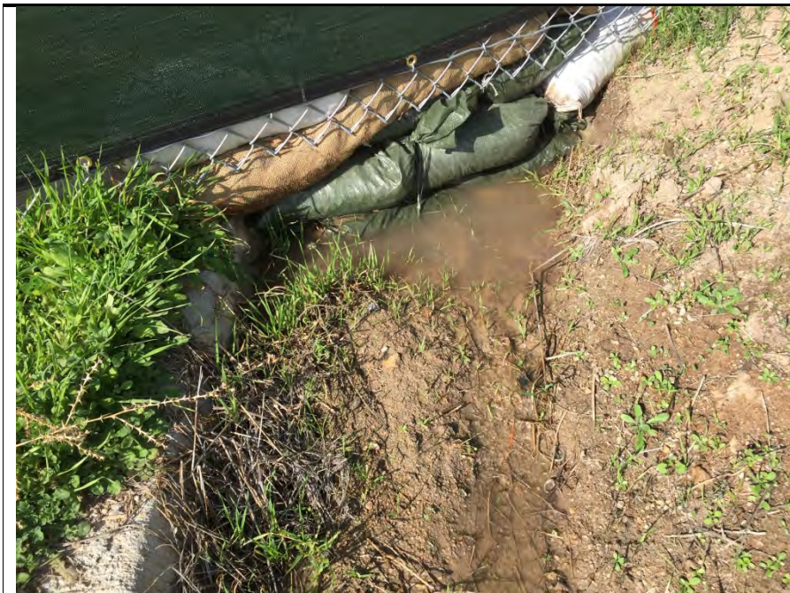
Photo 4: Outside of project limits where water seeped through the rock bags and wattle logs on December 12, 2016.
