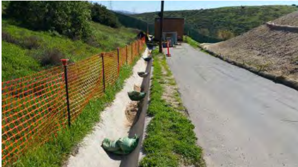
Caption Brow ditch near trailer has been cleared but for one wet area.
