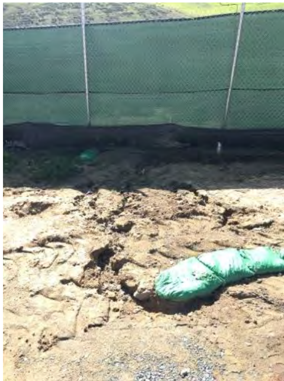
Caption Erosion near entrance, maintenance required
