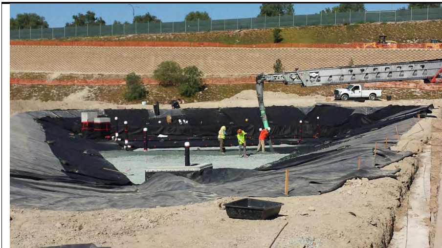
Photograph 2: Installation of the bio-retention pond base material during the week of October 15, 2016.
