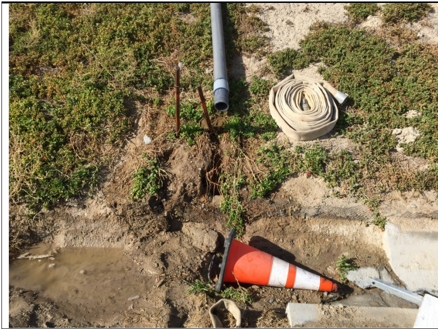
Photo 1: Recycled water pipeline where valve was pulled off pipe on December 12, 2016.
