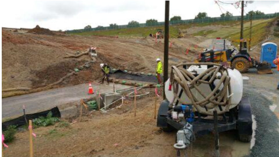
Caption Additional erosion BMPs installed in muddy entrance to substation.
