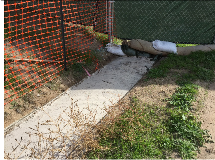
Photo 3: Last check dam prior at edge of project limits where spilled water backed up on December 12, 2016.
