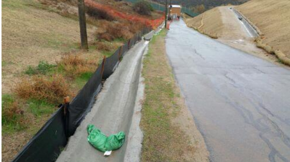
Caption Sediment capture on east brow ditch.
