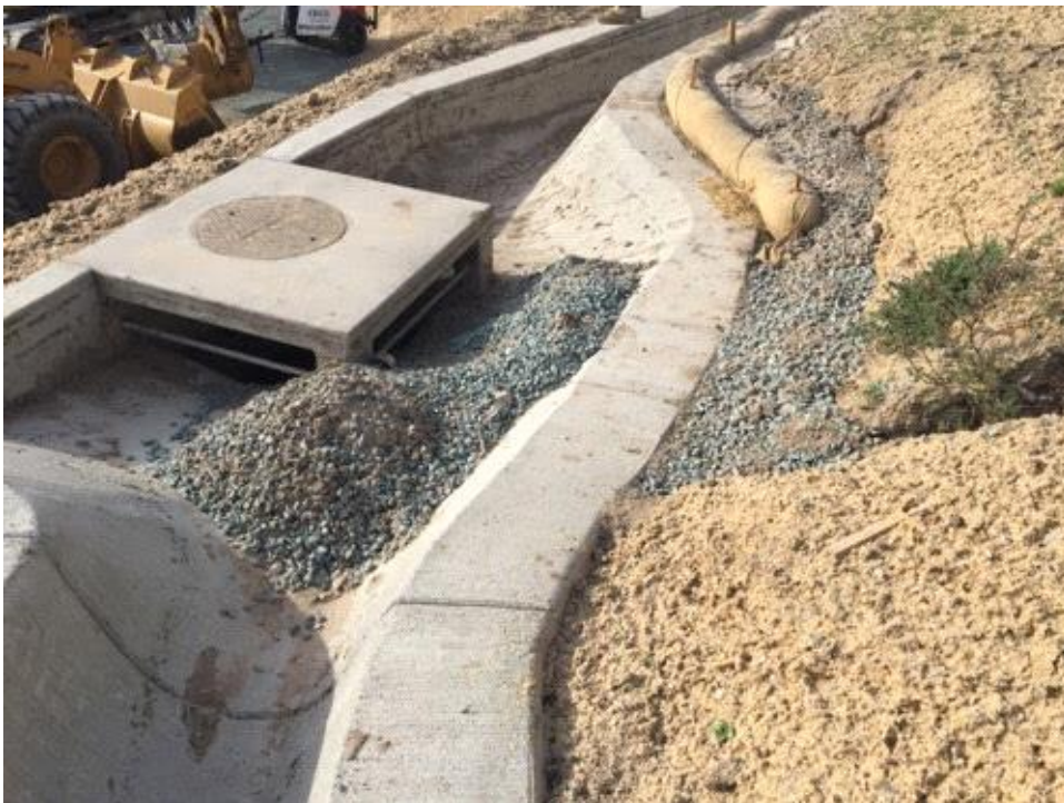
Caption Sediment and rock to be removed prior to storm event.
