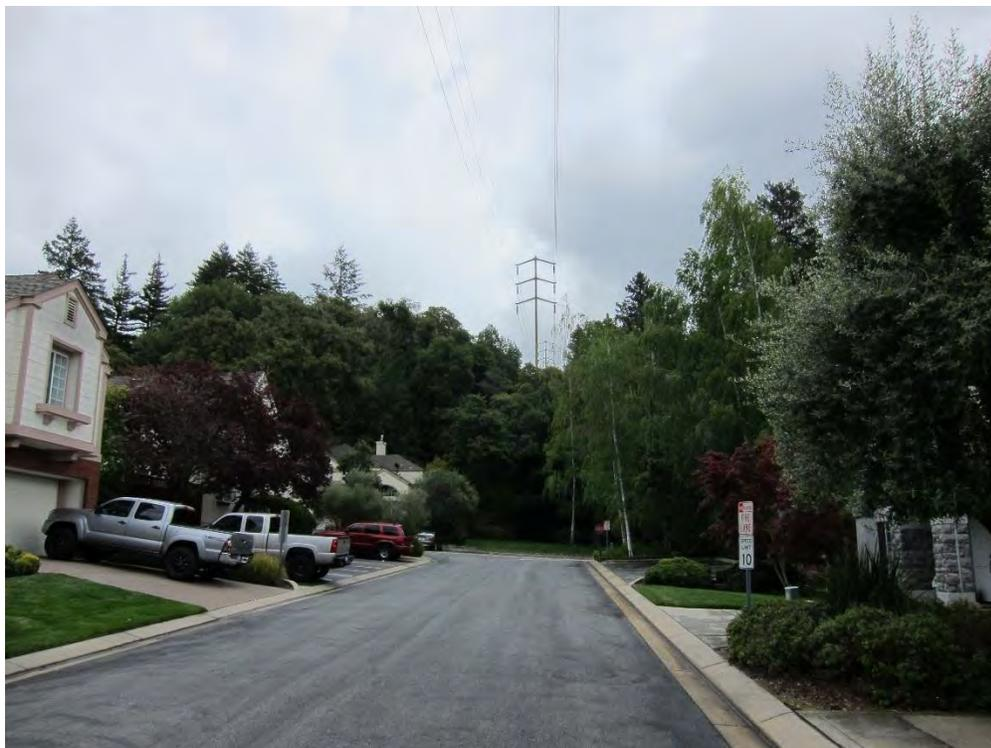
Photograph 11: Green Valley-Camp Evers Line – tubular steel pole (TSP) located south of Sidesaddle Circle in the City of Scotts Valley (approximately 80 feet in height)
