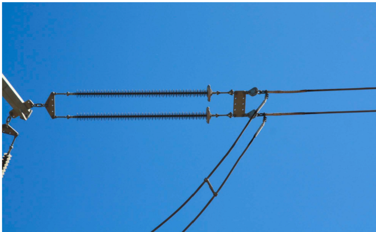
Figure 2.2-15 Representative Photograph of Bundled Conductor
