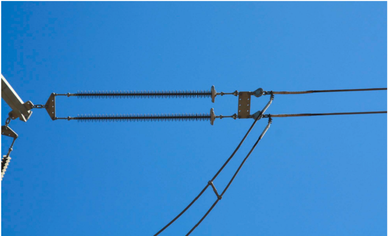
Figure 2.2-15 Representative Photograph of Bundled Conductor
