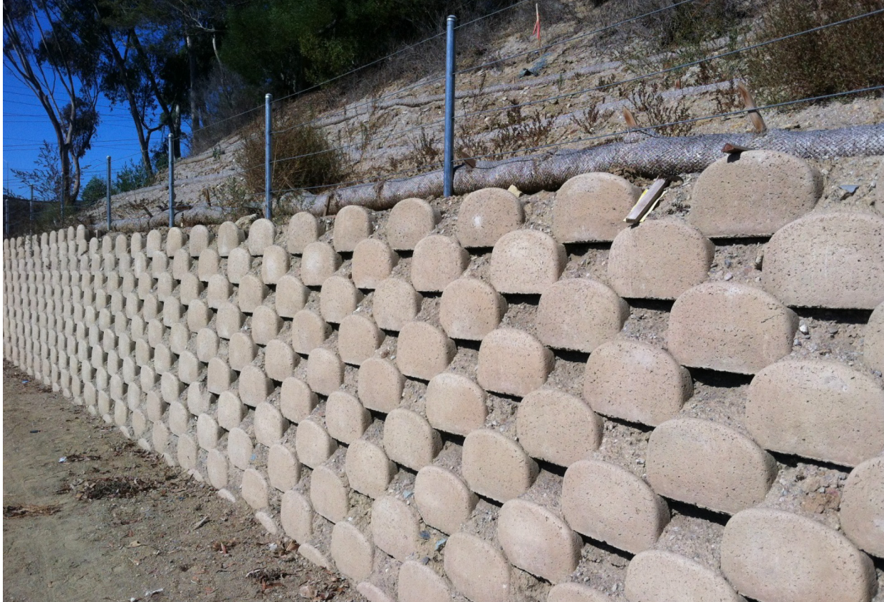
Figure 2.3-2 Typical Retaining Wall Face
