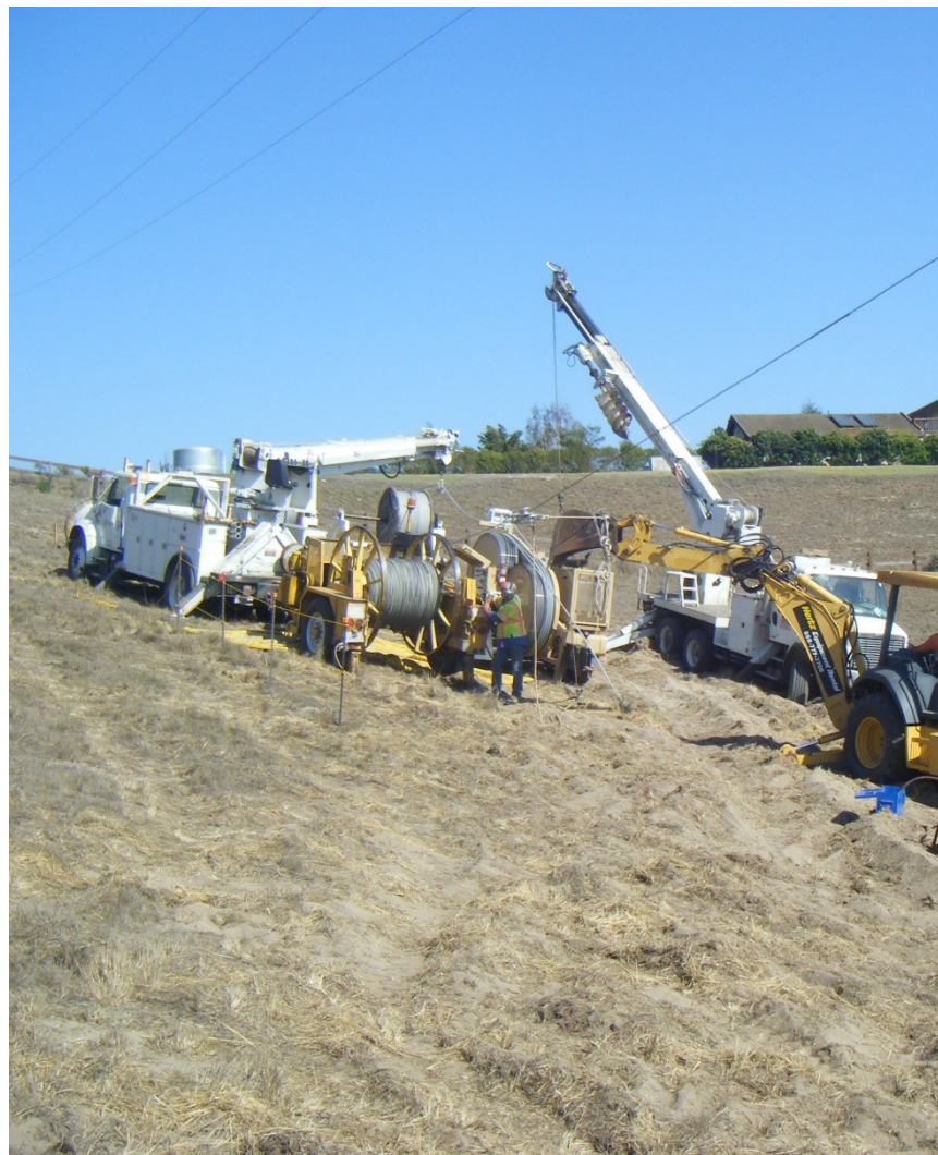
The cable reel and pulling rig are shown towed behind a line truck.
