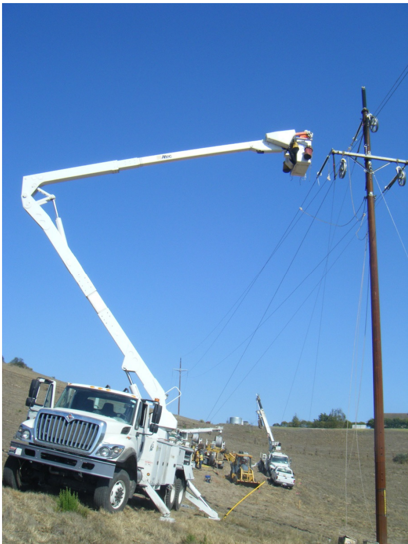
A bucket truck is shown in the foreground.
