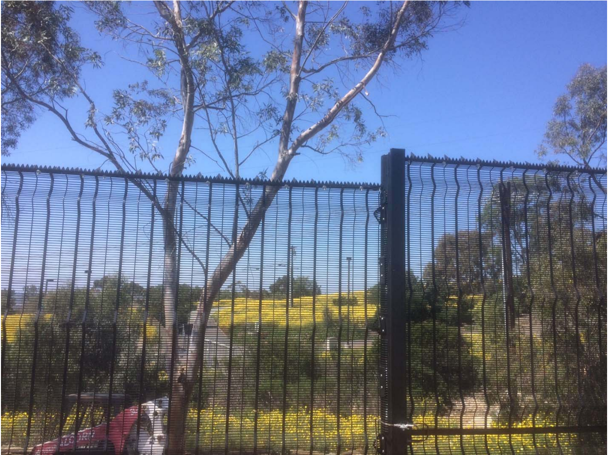
Example Photograph of Clear VU security fencing with Castle Spike anti-scale.
