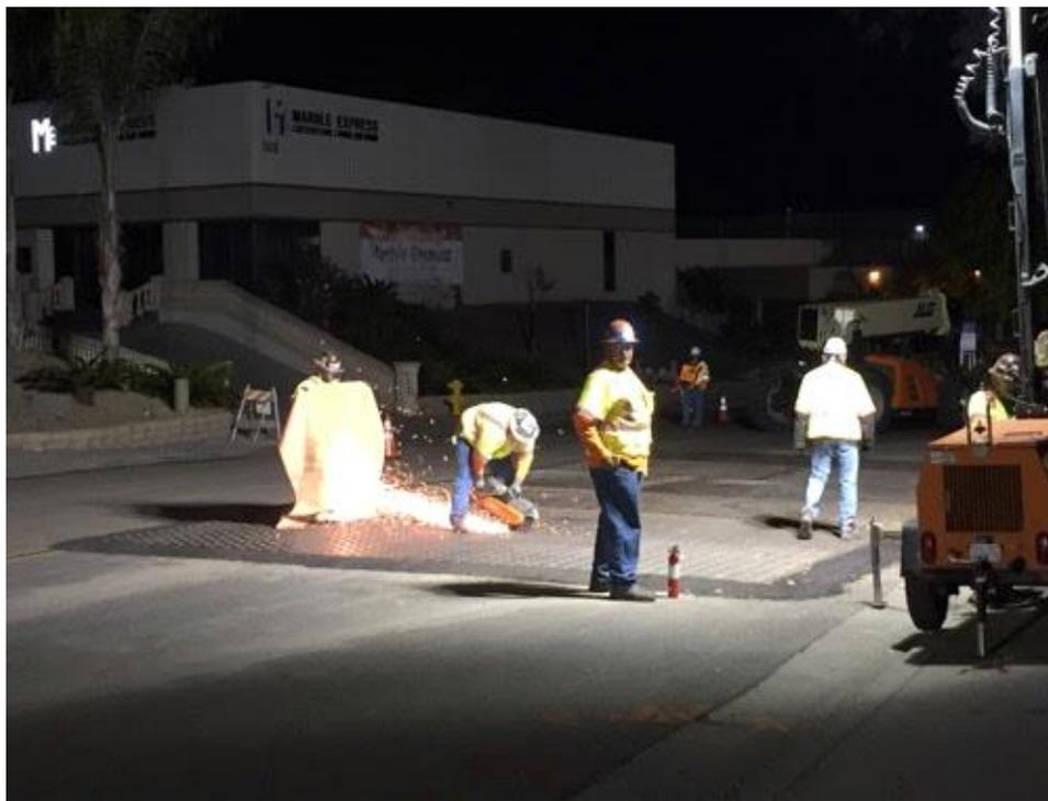
Caption Cutting asphalt with fire barrier in place.
