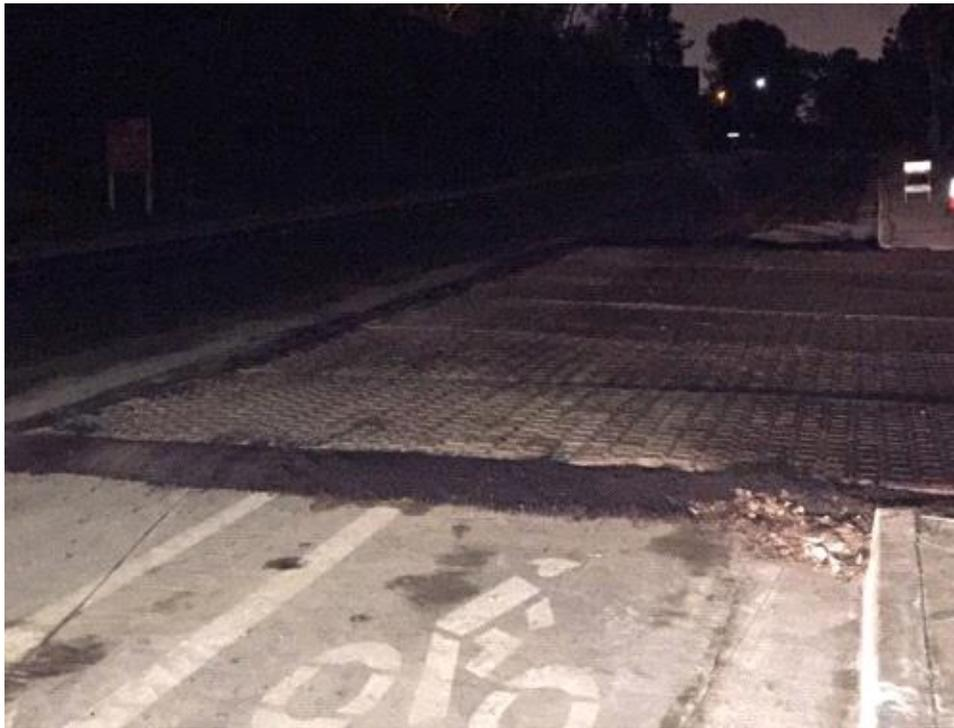
Caption Steel plates in place to cover trench. All sides patched with asphalt to seal the trench.
