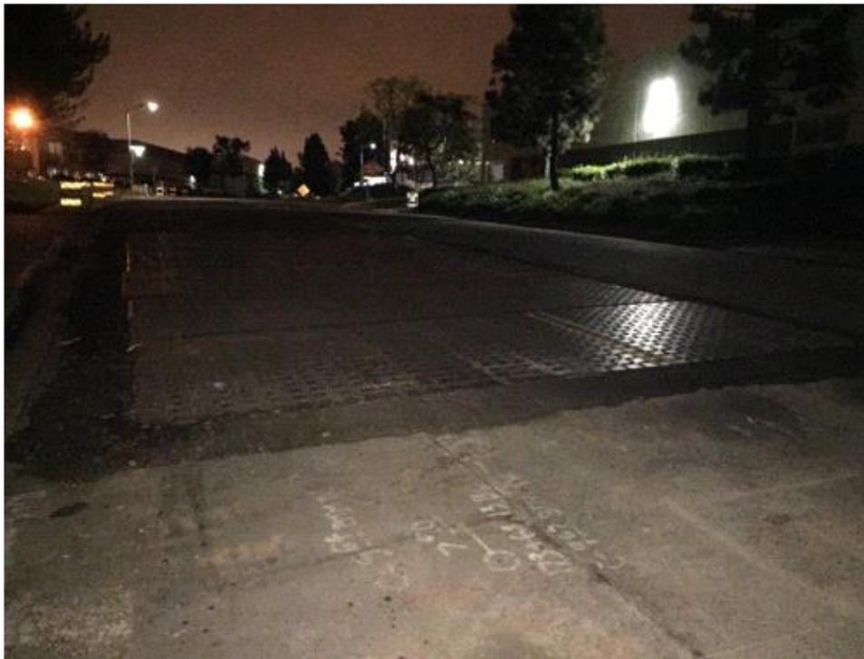
Caption Steel plates covering trenches and seams filled with asphalt to cover completely.
