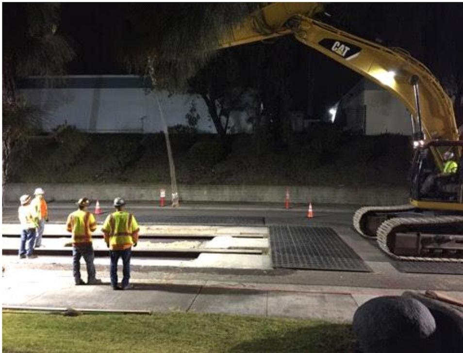
Caption Removing steel plates for shoring/ trench work.
