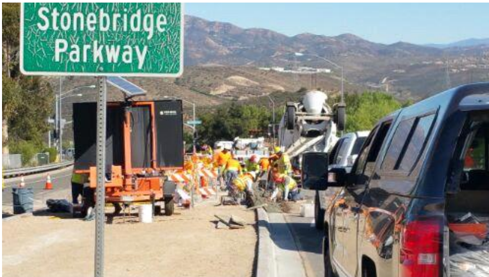
Caption Curb replacement, upper Pomerado Road.
