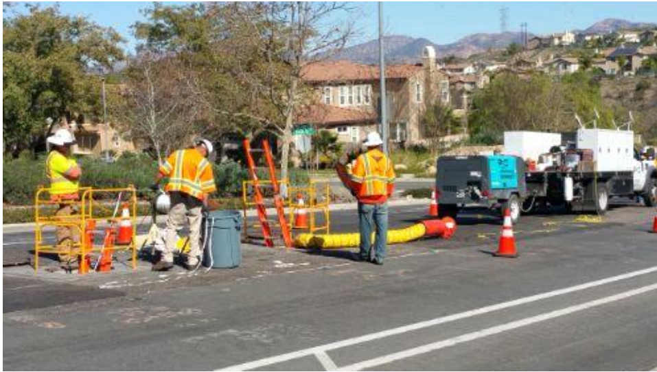
Caption Mandreling work area, Stonebridge Parkway.
