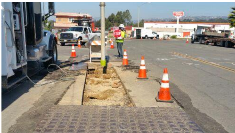
Caption Potholing site, Kearney Mesa Road.
