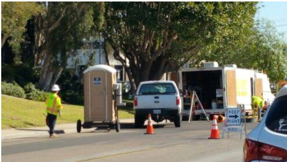
Caption Vault work area, Marilani Road.
