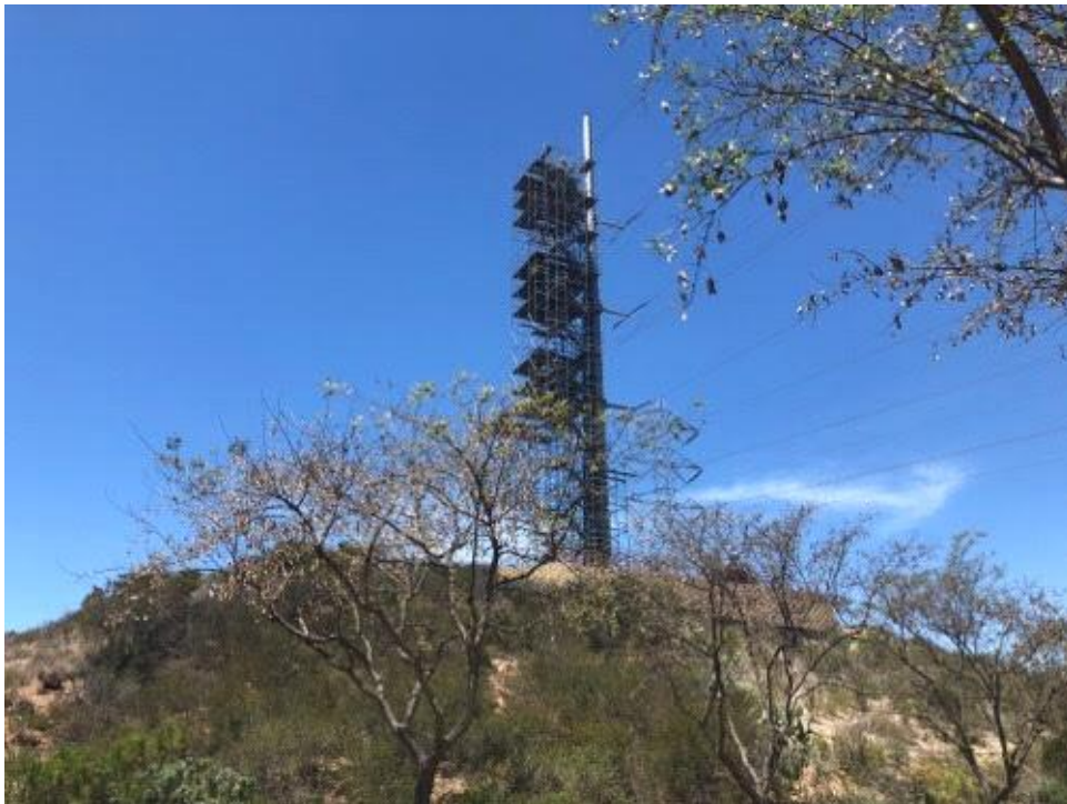
Caption P05 scaffolding.
