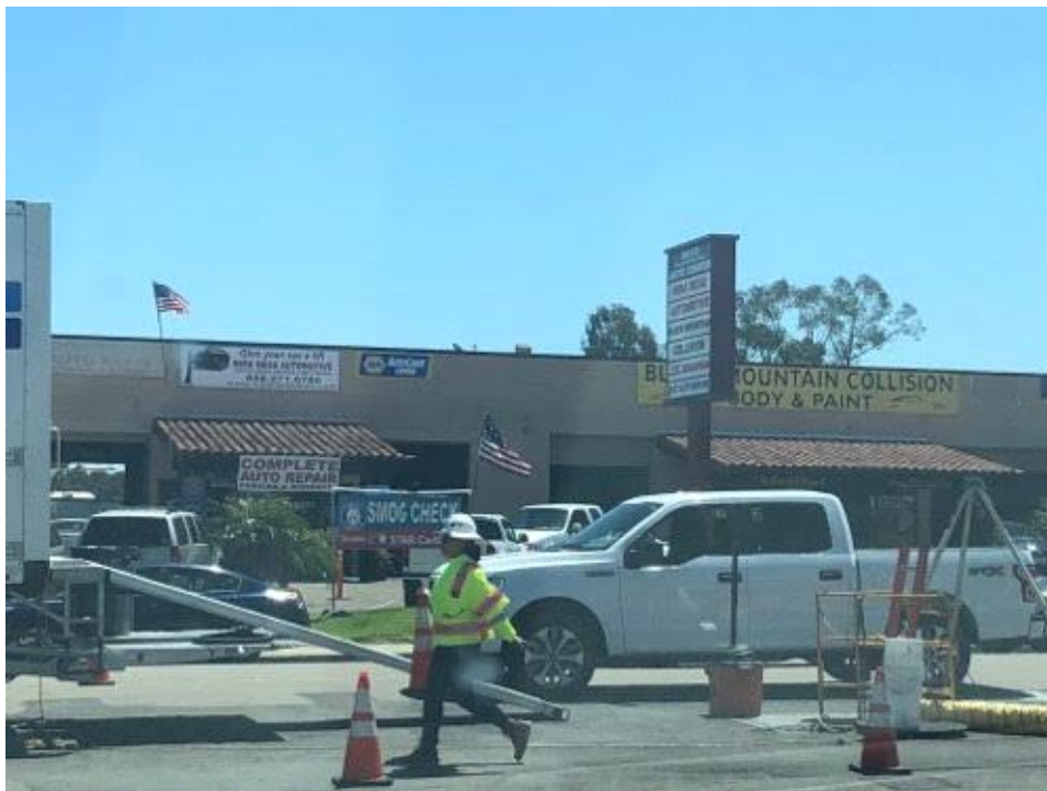
Caption Black Mountain Road vault work - traffic flowing normally.
