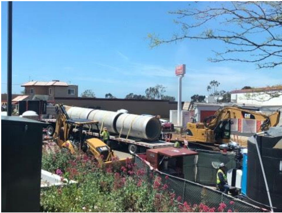
Caption Pipe delivery to west side bore pit.
