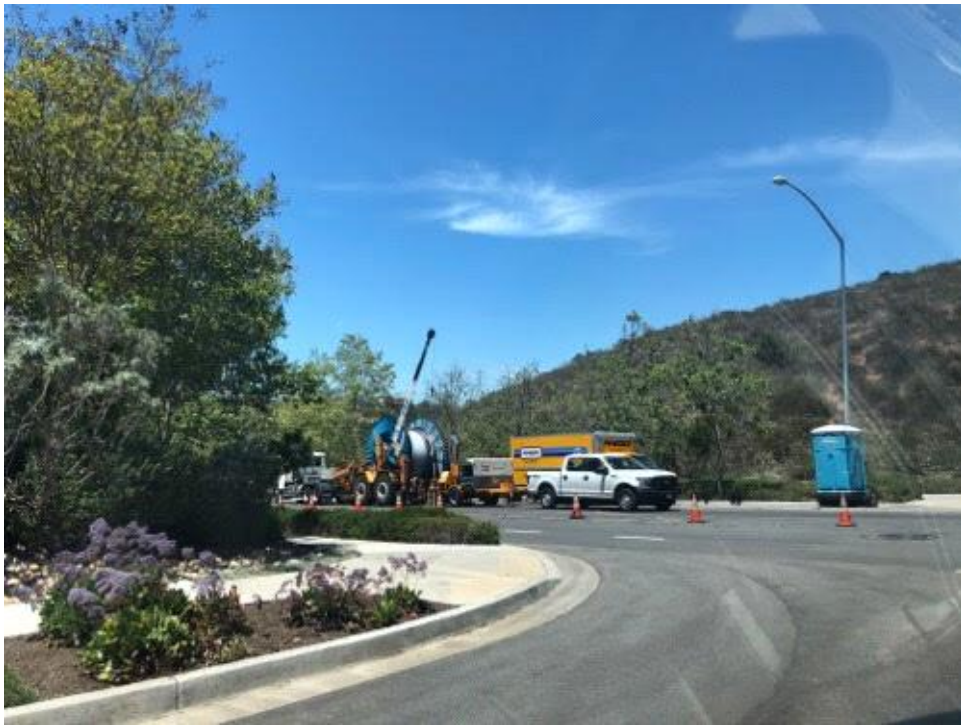
Caption Vault work on Stonebridge Parkway.
