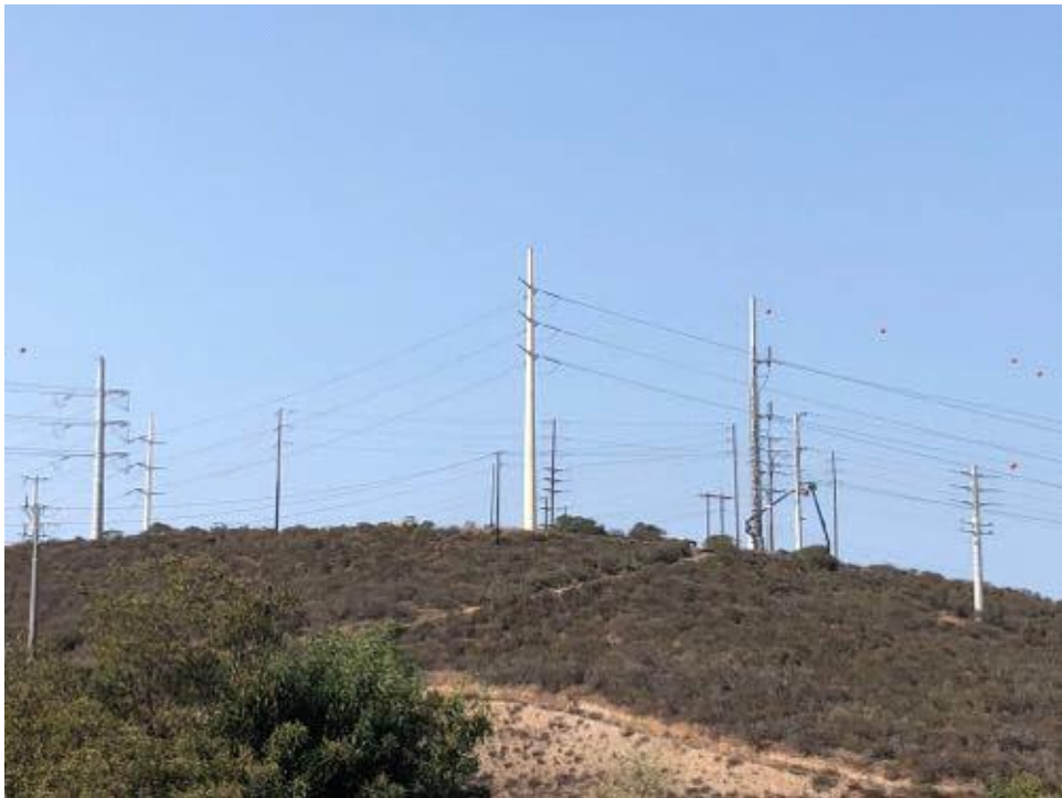
Caption Overhead work at P03.
