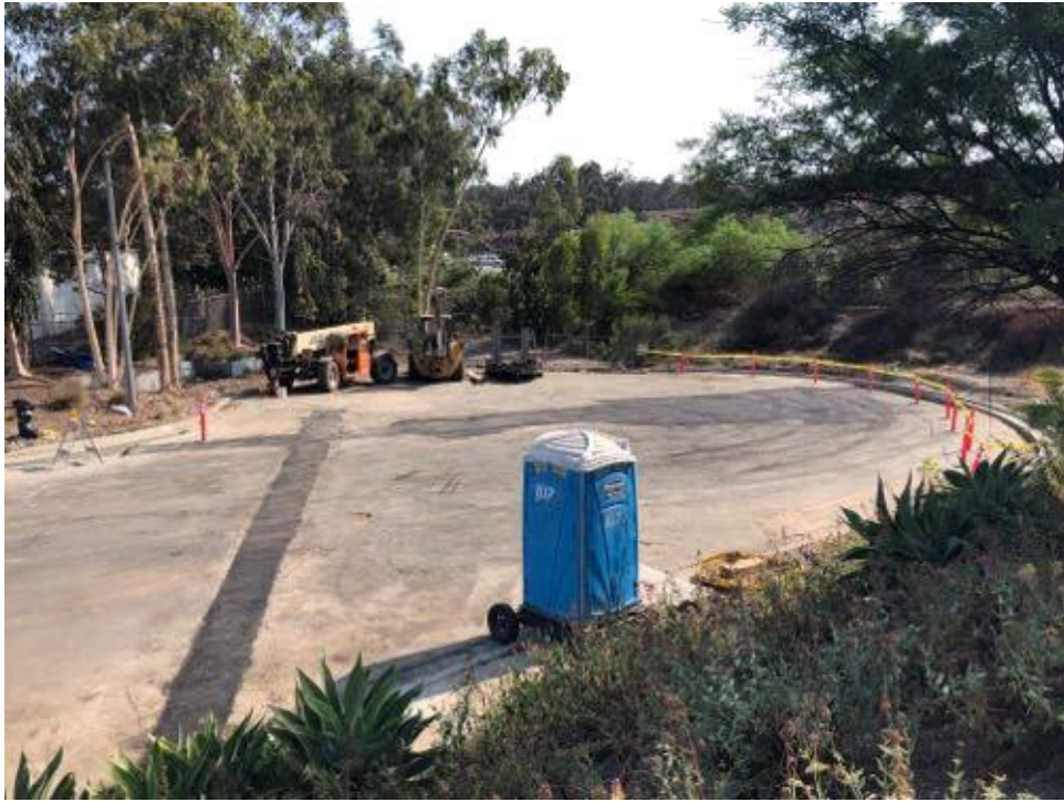
Caption Western bore pit closed up.
