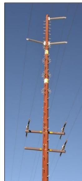
Example of a Weatherized Steel Replacement Structure
