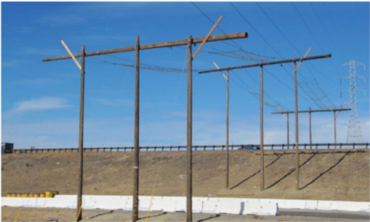
Example wood pole guyed guard structure with netting.
