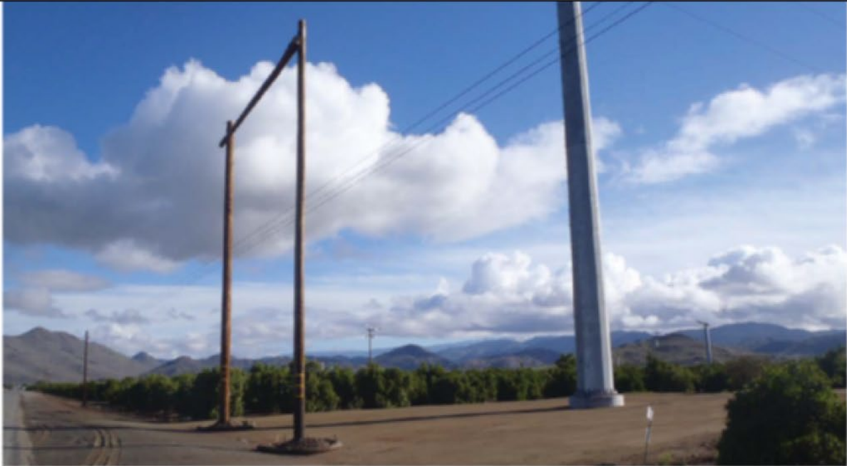
Example standard wood pole guard structure.
