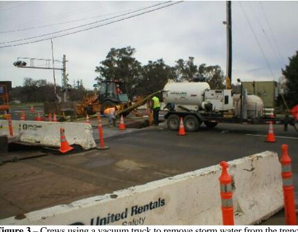
Figure 3 – Crews using a vacuum truck to remove storm water from the trench within Rocklin Road, January 30, 2006.
