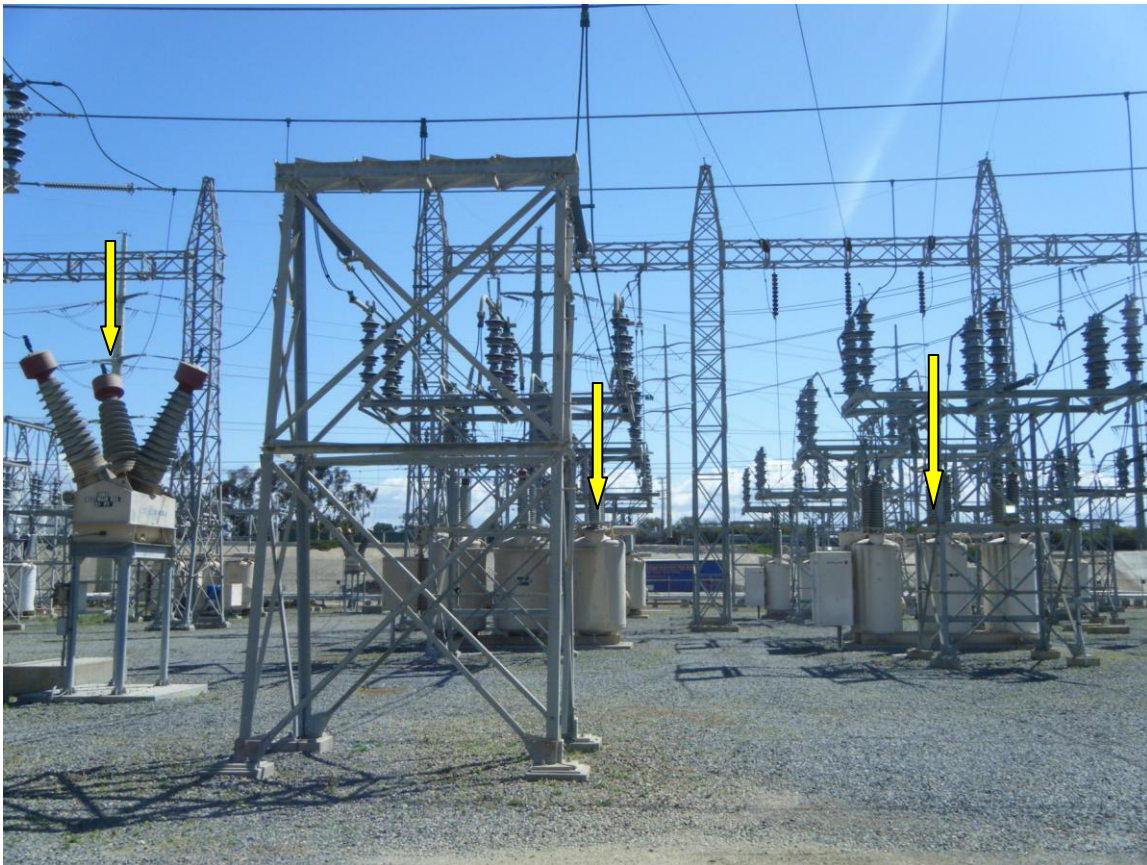
View facing east. Oil circuit breakers (examples located in middle of photo) will be replaced with gas breakers (example located on far left of photo).
