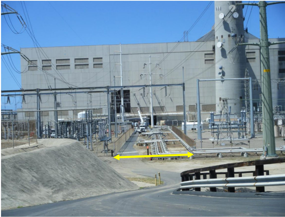
Area between 230-kV & 138-kV Switchyards. This area is 45-feet wide and includes a paved access drive, and below- & above-ground piping.
