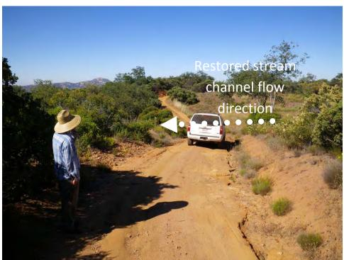
Figure C-22. View of same road crossing shown in Figure 23 at Site 11. Road cut areas will be filled to restore the natural topography surrounding the stream channel valley.
