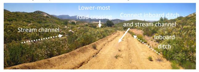
Figure C-12. At Site 1 looking down-gradient along the roadway with the stream channel running parallel to the left and an inboard ditch running on the right. The inboard ditch connects the abandoned road/ditch channel upstream to the ditch channel downstream.
