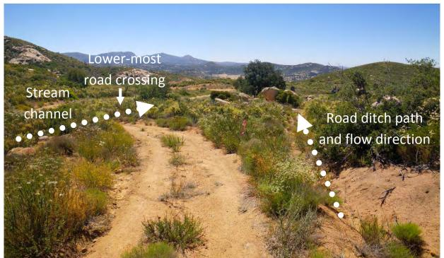
Figure C-13. At Site 1 looking down-gradient along the roadway with the inboard ditch diverting away to the right and the stream channel crossing on the left.
