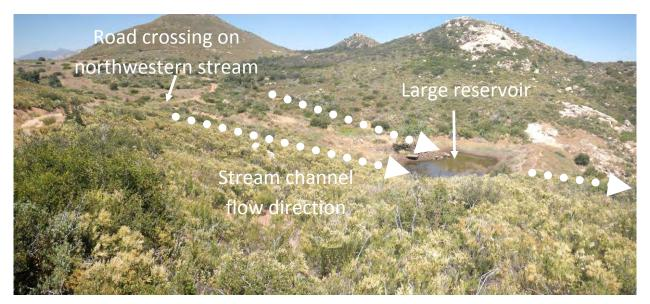
Figure C-25. Eastward view of the large reservoir, dam, road crossing, and northwestern and northeastern stream channels at Sites 2 and 3. Removal of road crossing and pond storage berms and lowering of the large reservoir dam will enhance hydrologic connectivity from the headwaters to the downstream of the large reservoir.
