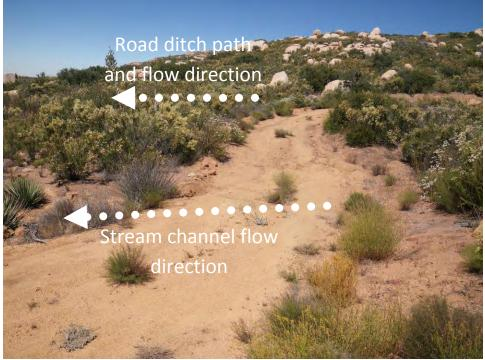
Figure C-14. At Site 2 looking at the lower-most road crossing of the stream channel that drains to the southwest meadow. The road ditch is also shown here.
