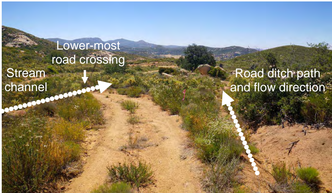
Figure 20. At Site 2-A looking down-gradient along the roadway with the inboard ditch diverting away to the right and the stream channel crossing on the left.
