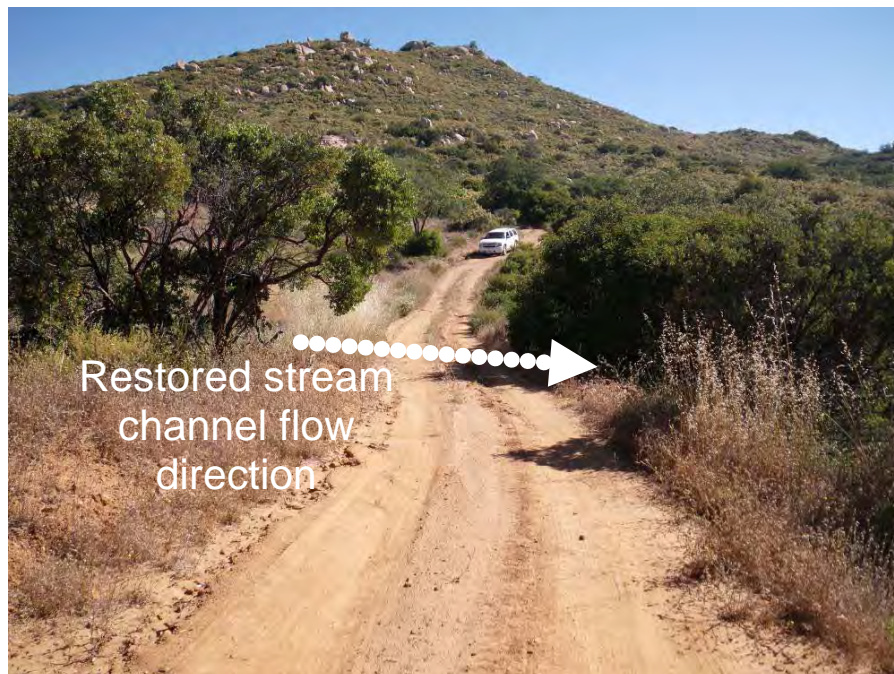
Figure 26. View of existing road crossing at Site 11. Removal of road will re-connect the upstream and downstream reaches of this ephemeral stream channel, in addition to re-focusing the headwater drainage to the stream channel.
