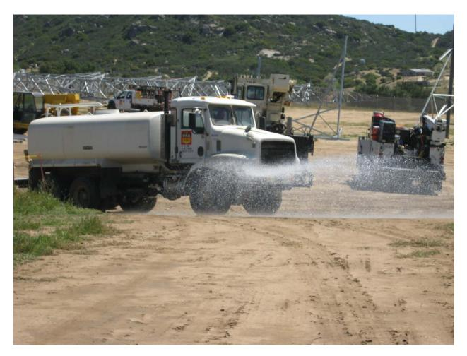
Controlling dust with the water truck at Bartlett/Hauser Creek Construction Yard, 4/27/2011.
