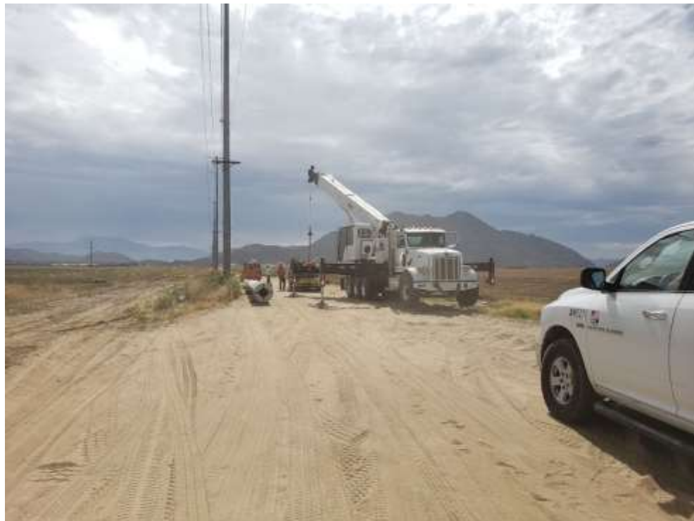
Photo 2 – Staging poles off Menifee Road and Construction Area UNK 250 (August 6, 2019).
