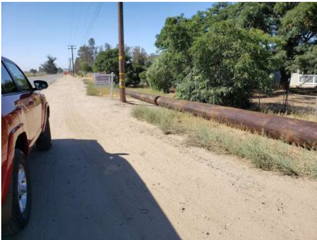
Photo 4 – Wood poles staged at construction areas that were not released for construction (August 20, 2019).
