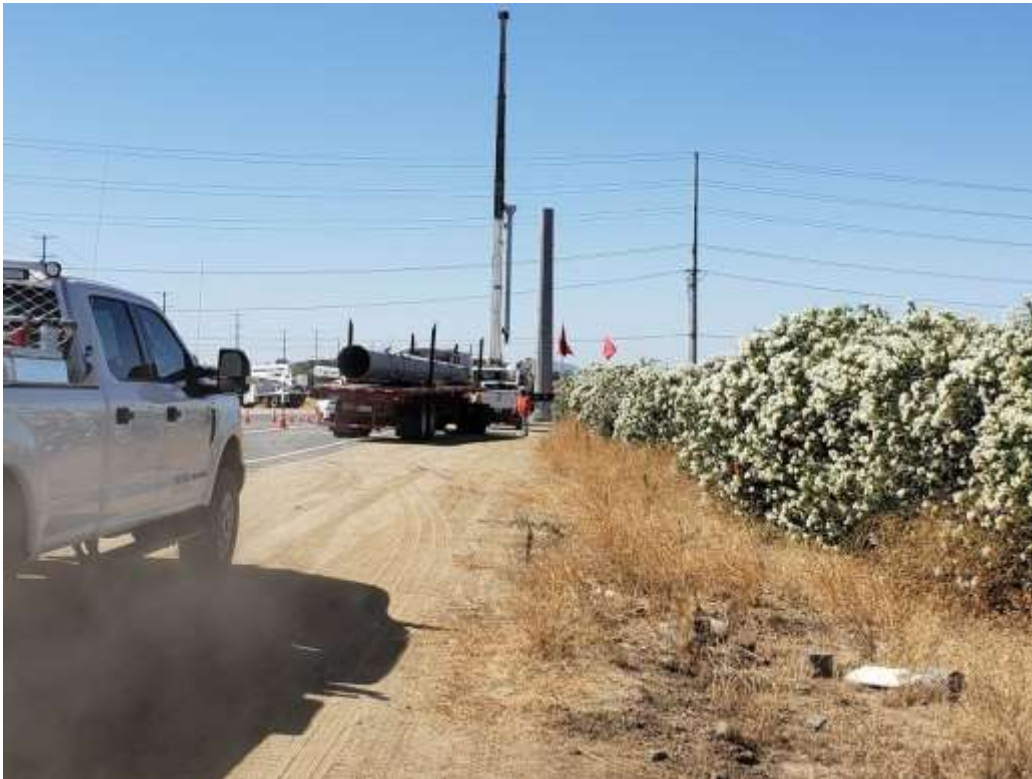
Photo 3 – Pole installation at Construction Area UNK 247 (August 12, 2019).
