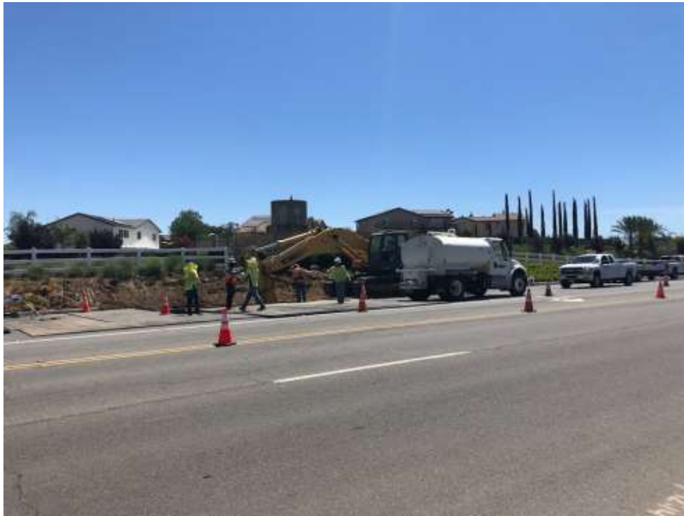
Photo 1 – Vault excavation for the southern underground on Leon Road (August 16, 2019).
