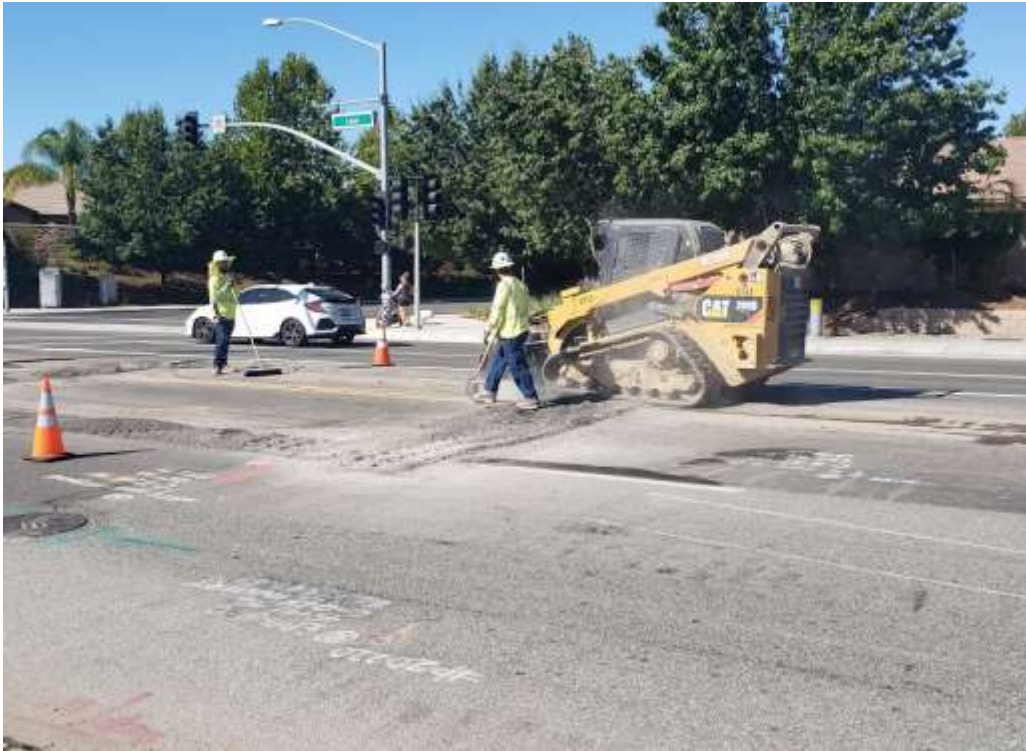
Photo 1 – Construction activities on the southern underground (September 17, 2019).
