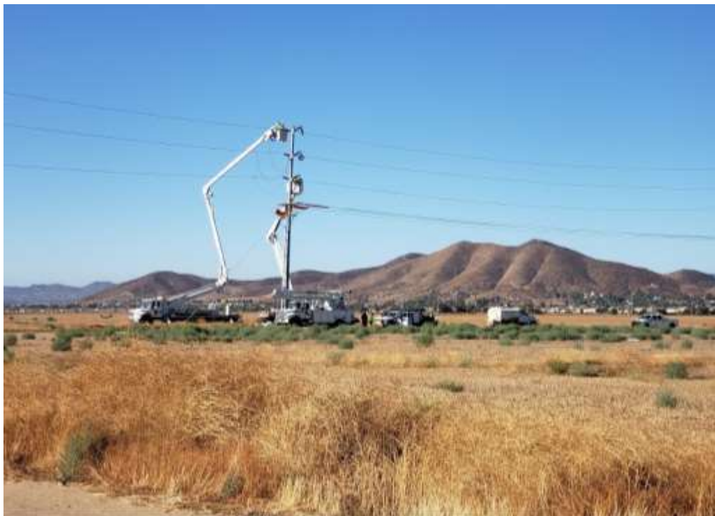
Photo 2 – Reconducting activities from Construction Area UNK250 to UNK01 (September 17, 2019).
