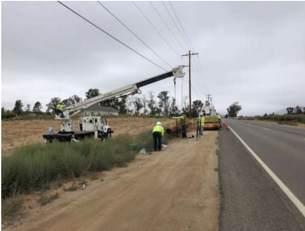
Photo 3 – Framing pole 2150098E at Construction Area UNK171 (September 5, 2019).
