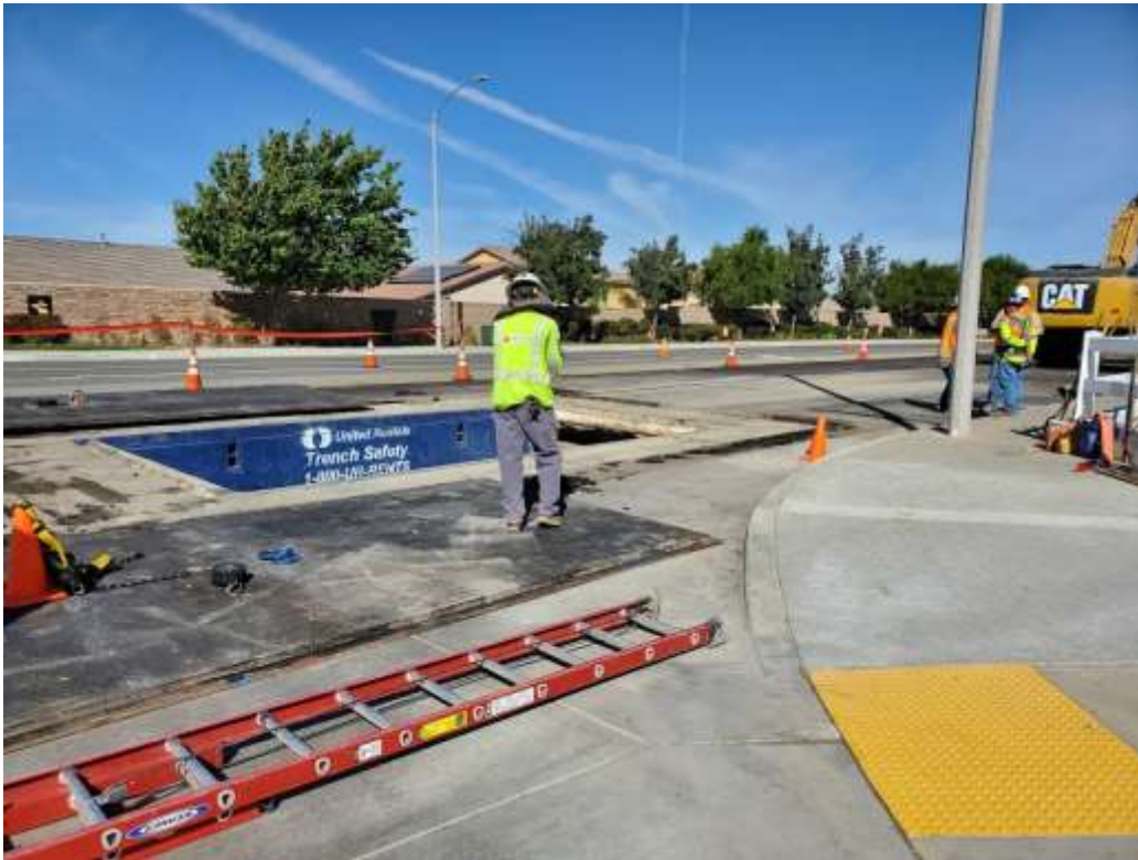
Photo 1 – Construction activities at Vault 3B on the southern underground (October 16, 2019).
