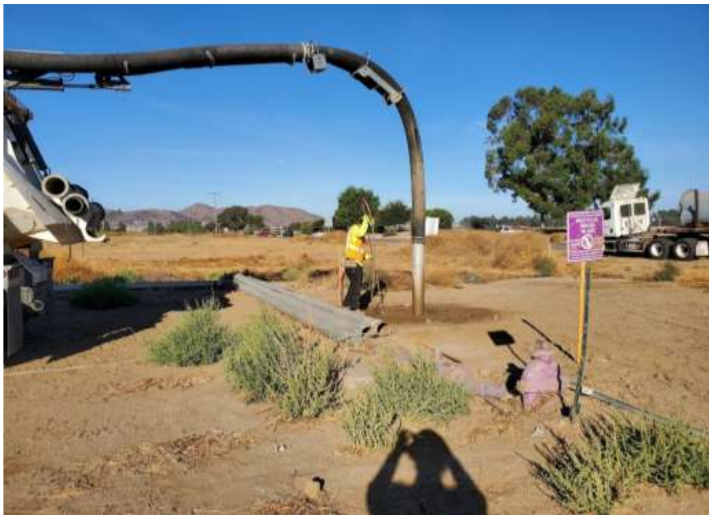
Photo 2 – Hydrovac drilling activities at Construction Area UNK20 (October 16, 2019).
