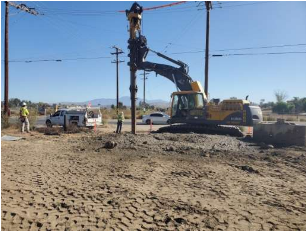
Photo 3 – Drilling at Construction Area UNK155 (October 23, 2019).
