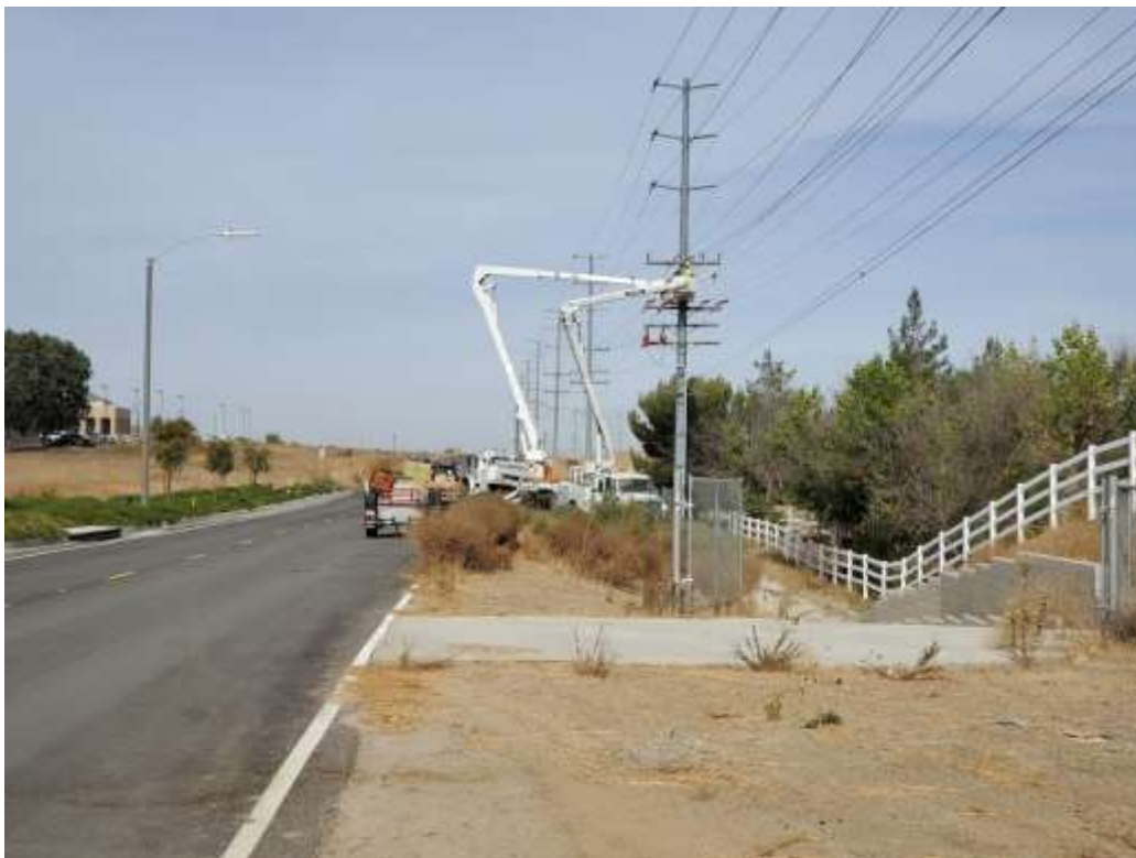
Photo 4 – Reconductoring activities at pole 4402009E, Segment 2 (November 13, 2019).
