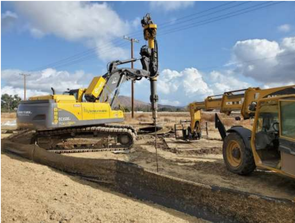
Photo 3 – Foundation activities at Construction Area UNK40, Segment 1 (November 20, 2019).
