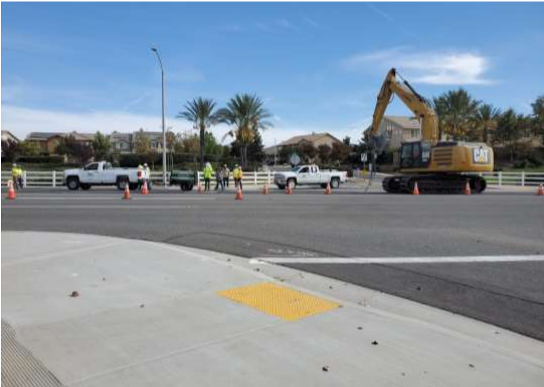
Photo 1 – Construction activities on the southern underground (November 13, 2019).
