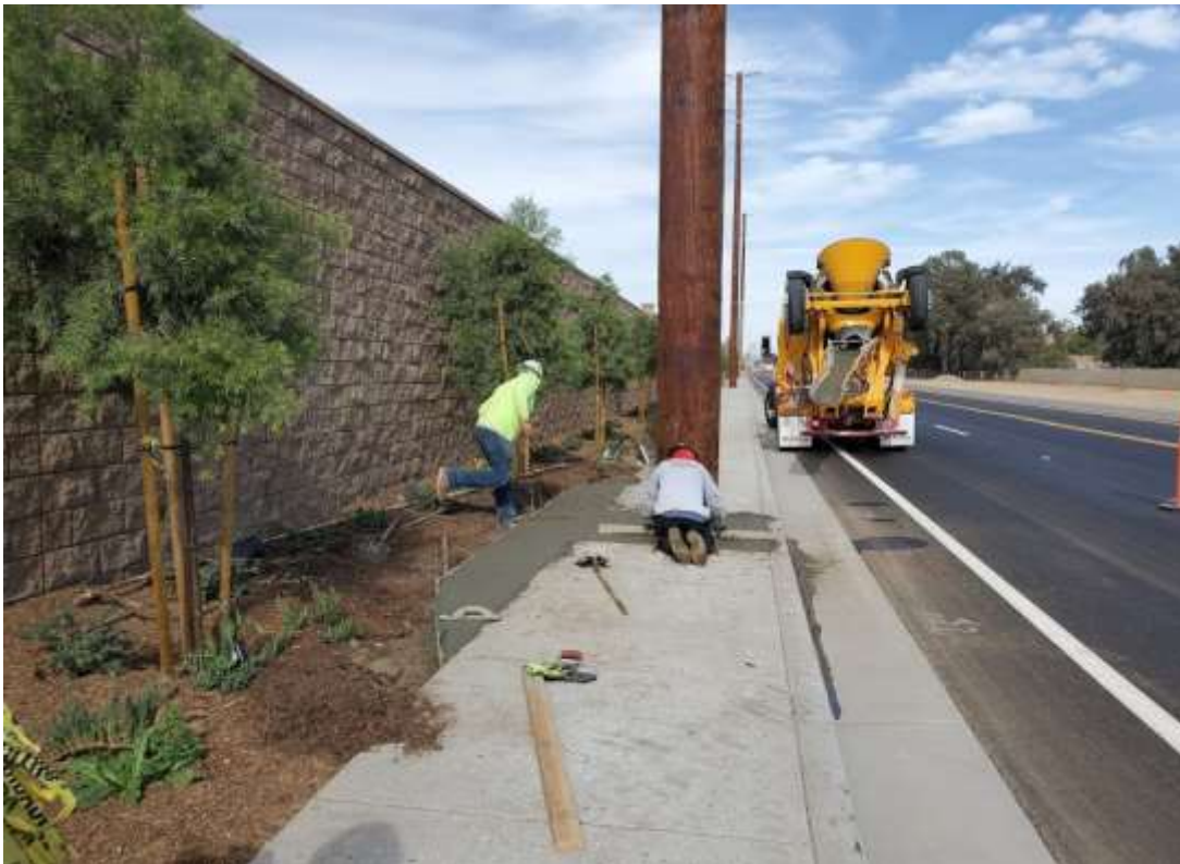
Photo 2 – Sidewalk repair at Construction Area UNK194, Segment 1 (November 13, 2019).
