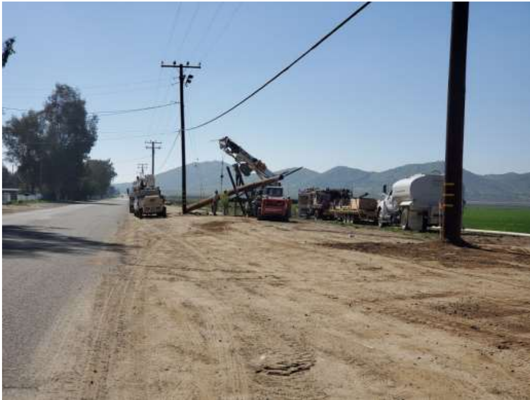
Photo 1 – Setting wood pole at Construction Area UNK23 (February 19, 2020).
