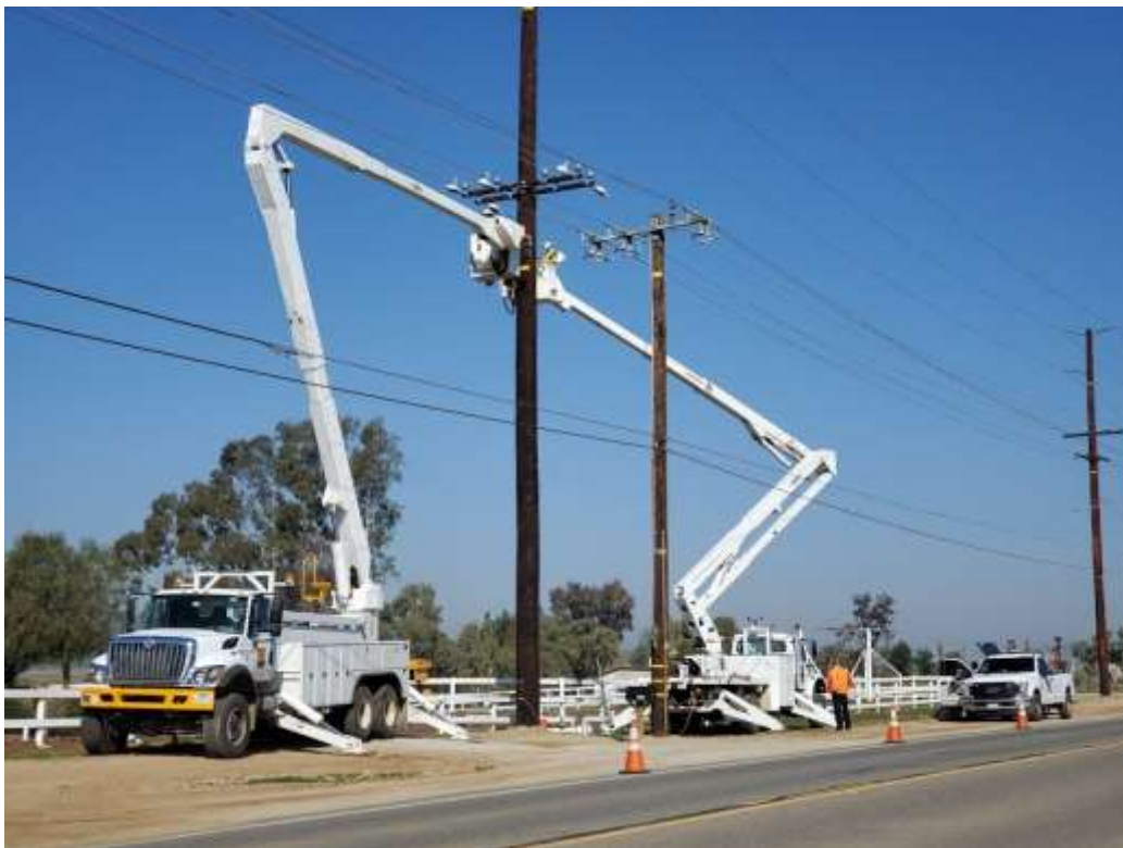
Photo 2 – Distribution activities at Construction Area UNK159 (February 19, 2020).
