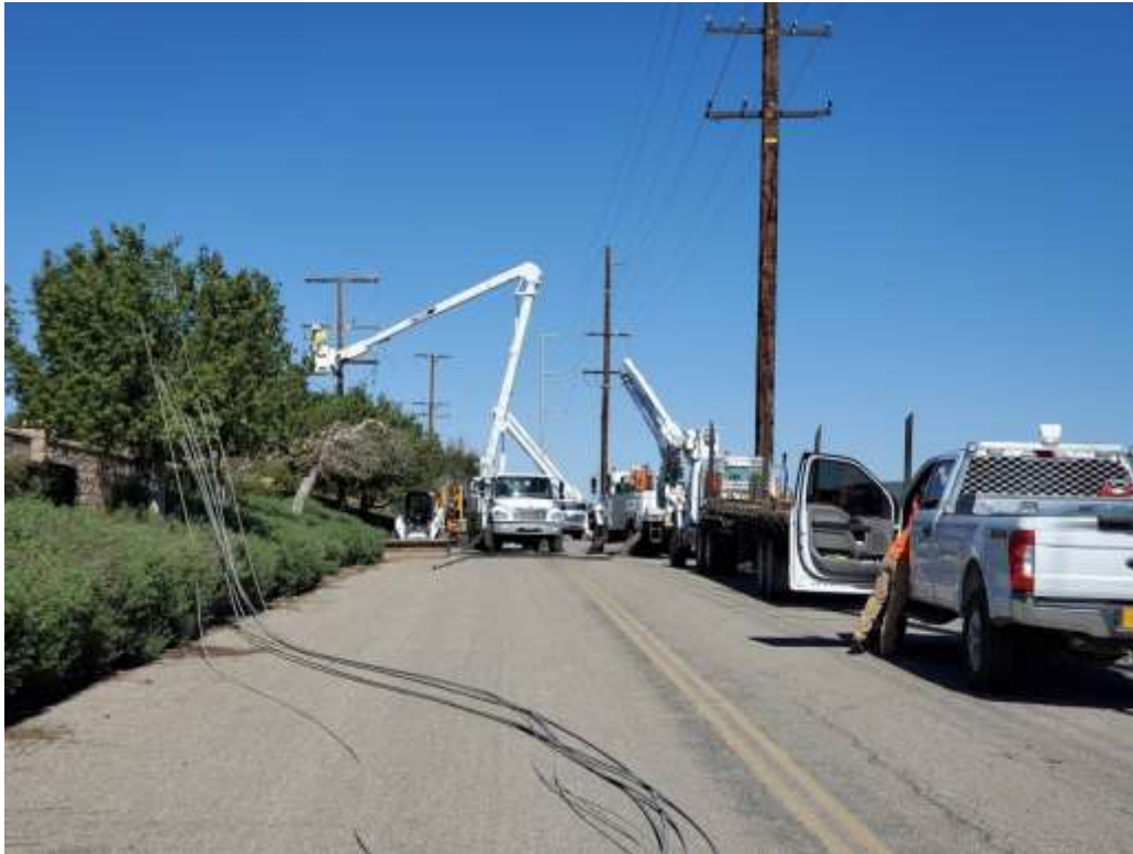
Photo 3 – Distribution cutover construction activities at UNK224 (February 25, 2020).
